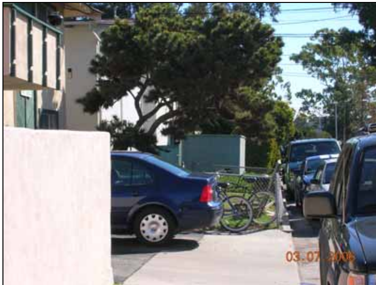
Existing Conditions along Sabado Tarde Road
