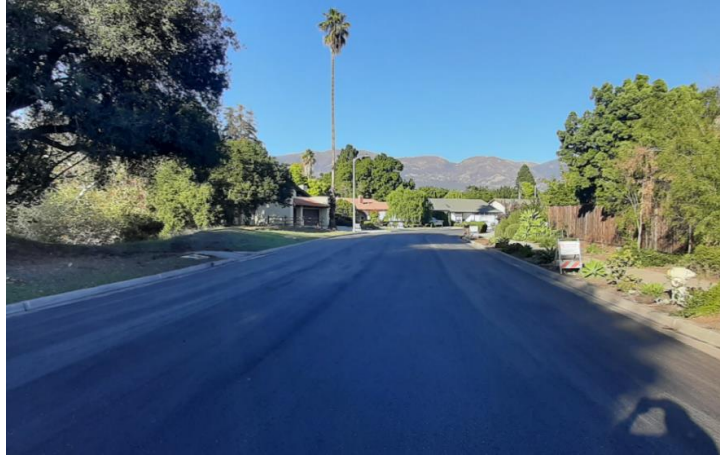
Figure 1: 2021-2021 Countywide Pavement Rehabilitation and Fog Sealing
