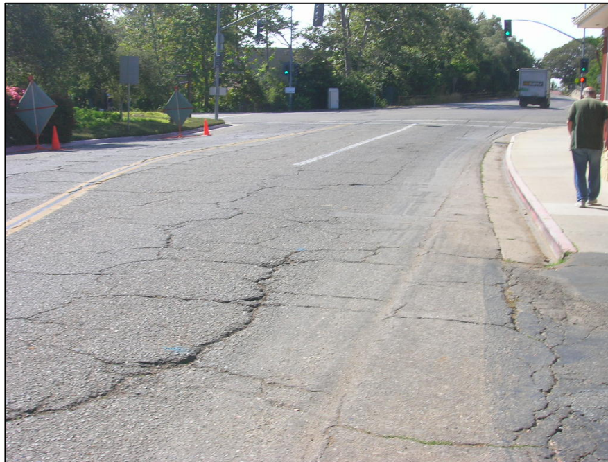
San Ysidro Rd, typical to be rehabilitated.
