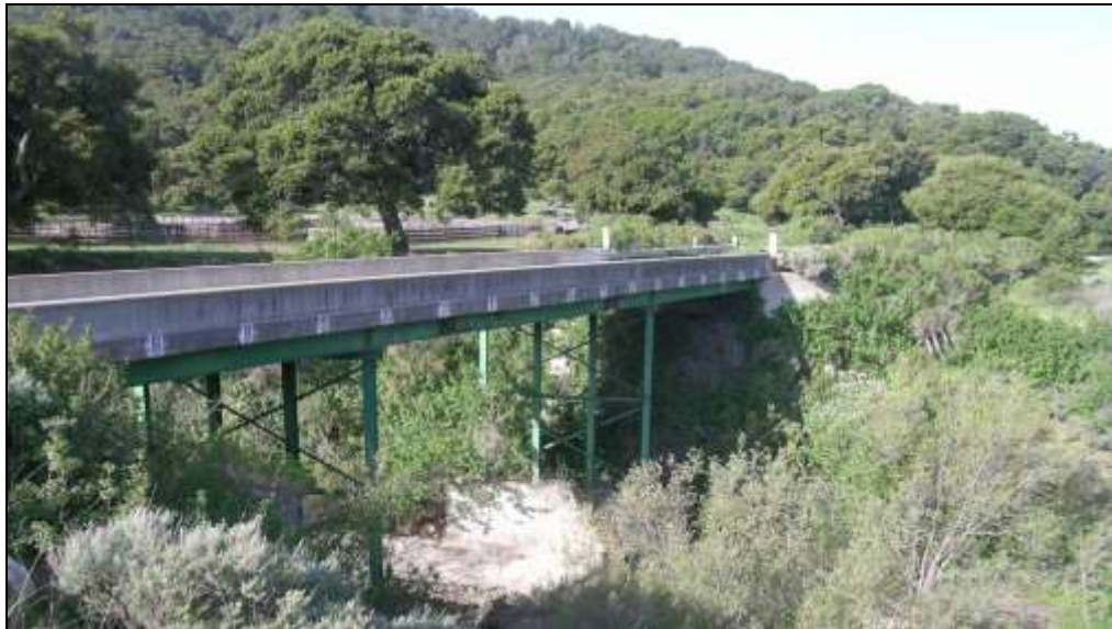
Jalama Road Bridge No. 51C-0017 from the northeast, looking upstream
