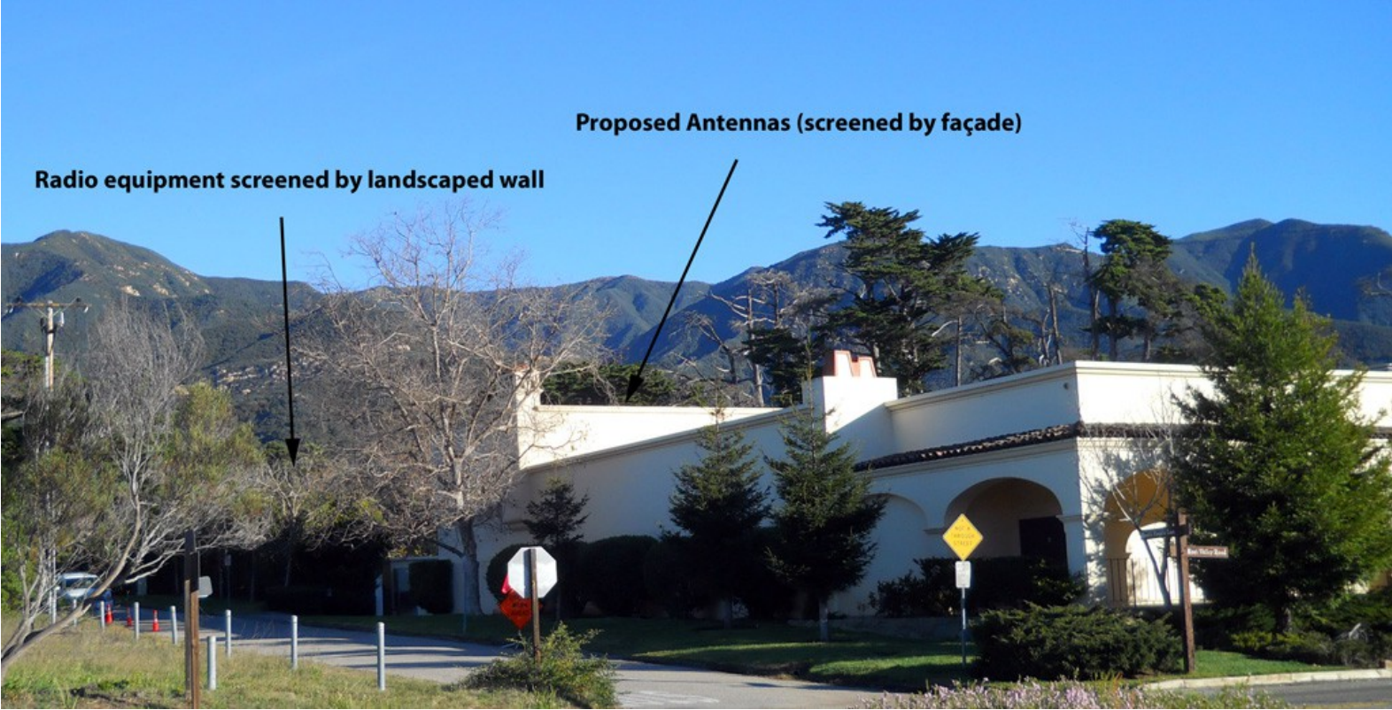
Photograph of the Approved Facility viewed from the southwest
