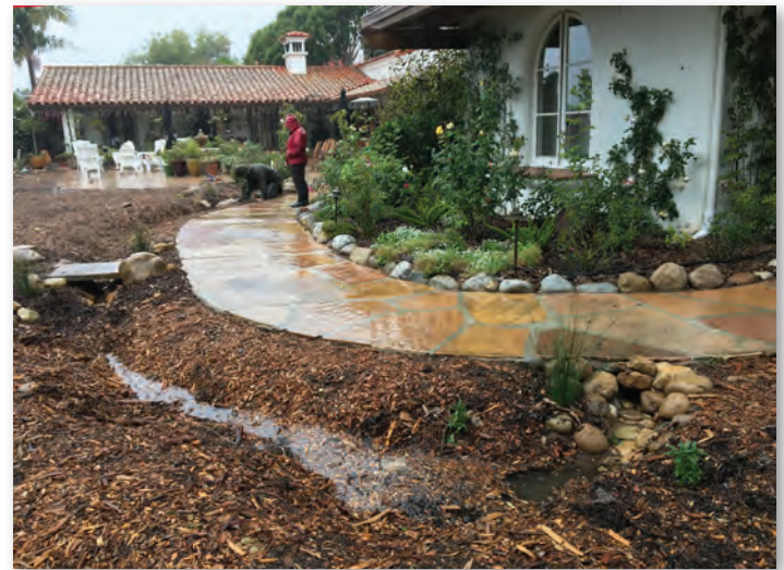
A swale infiltrates rooftop rainwater from the downspout at right and the walkway. Rainwater infiltration should be sited at least 8 ft from the foundation.
