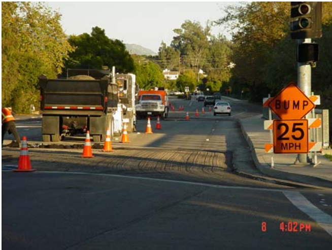
Polyester Concrete Overlay
