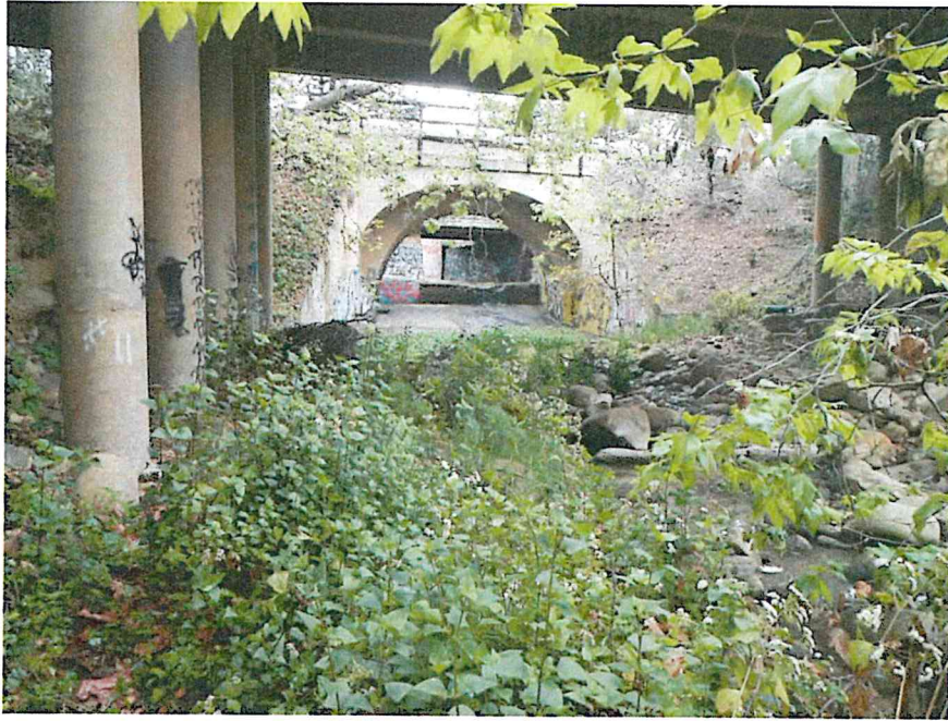
Photo 1. View of Toro Canyon Creek from south of Bridge 51C-063.
