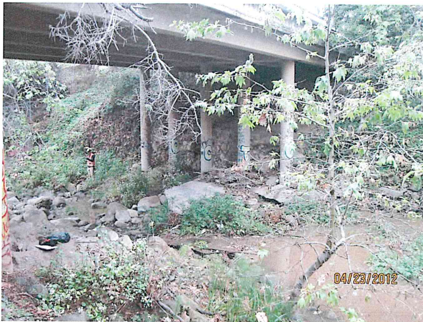
Photo 4. View of Toro Canyon Creek and Bridge 51C-063, looking southwest.
