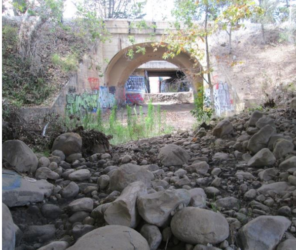
Upstream view under Bridge 51C-163
