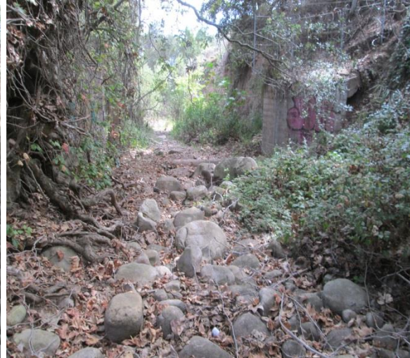
Downstream view under Bridge 51C-163
