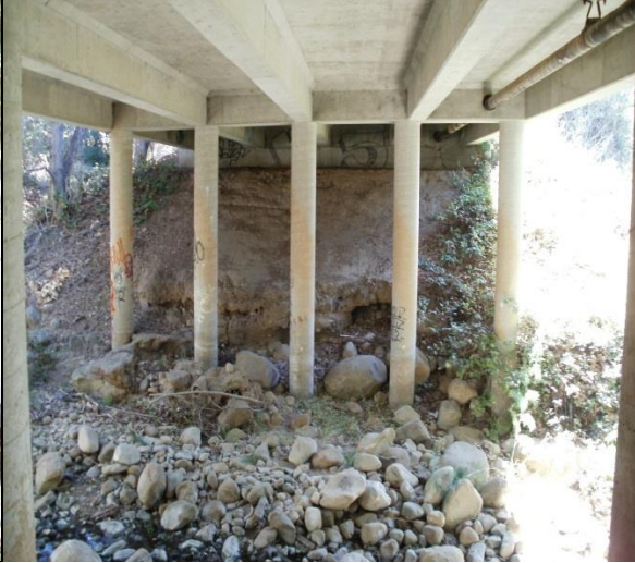
Eastern side creek channel view
