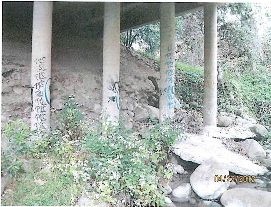
Photo 3. View of west abutment and piers of Bridge 51C-063.
