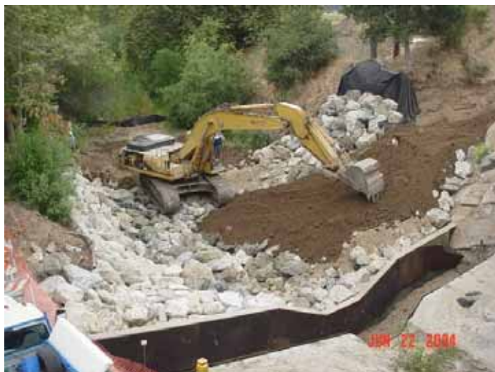
Adding Rock Slope Protection
