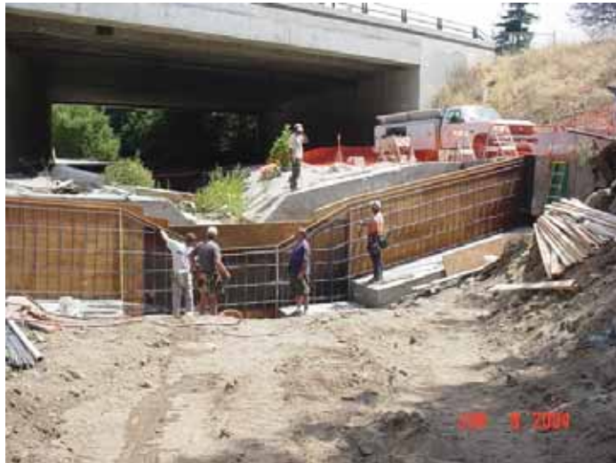
Construction of Retaining Wall
