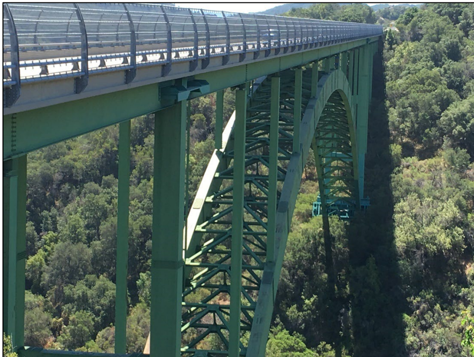
2. View of Cold Spring Canyon Bridge with 2012 barrier installed.
