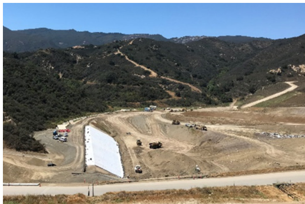
Liner System Installation for Phase IIIC GWPS Project
