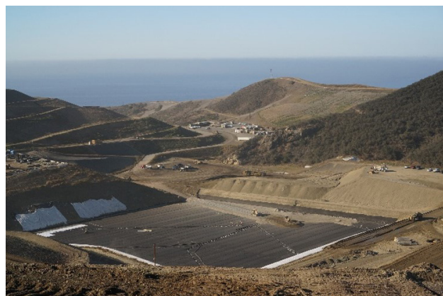
Liner system installation of Phase IIIB GWPS Project
