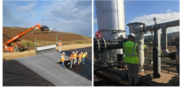
Liner system and landfill components installation during Cell I construction.
