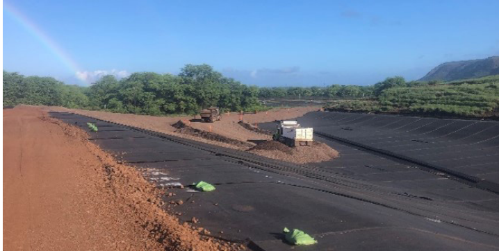
Liner system installation during Cell II construction.
