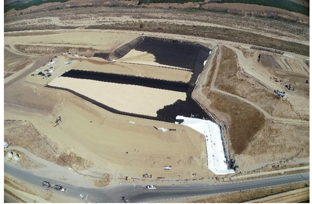
Liner system installation for the Cell 1 Phase 1 Extension Liner Project
