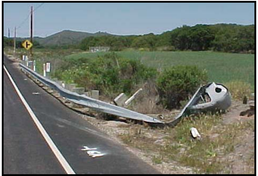
Photo: Damaged Terminal System
