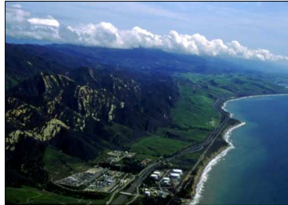
Gaviota Oil and Gas Processing Facility - Wm. B. Dewey
