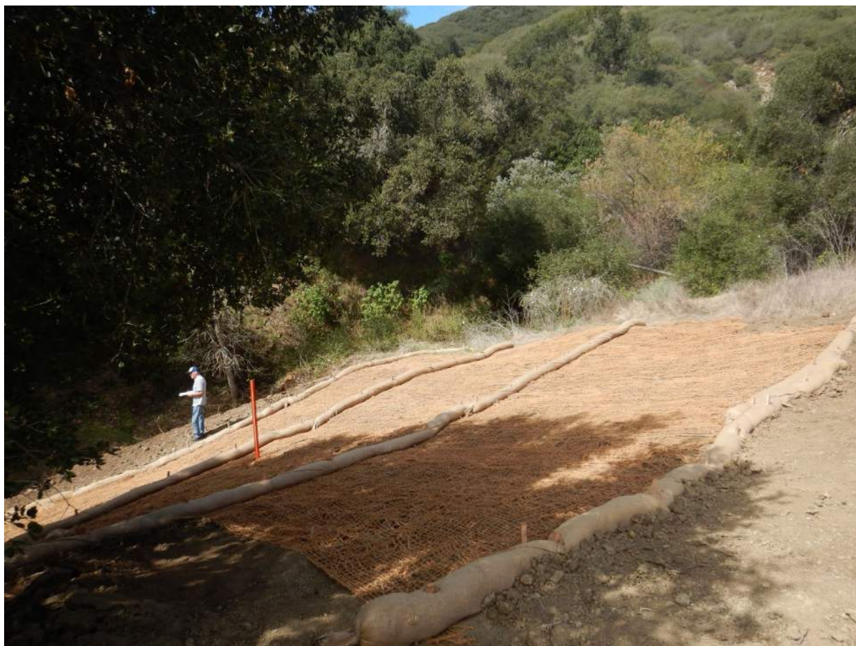
Figure 28. Loose soil with inadequate jute netting and waddles applied to only a portion of the ground disturbance. Orange stake site of pipeline anomaly repair site.
