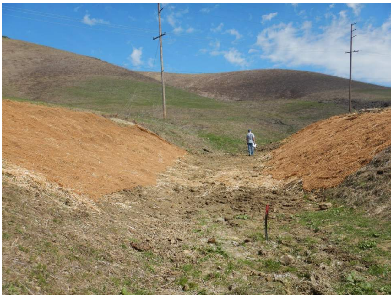
Figure 24. Orange painted stake marks the point of in-channel pipeline anomaly repair.
