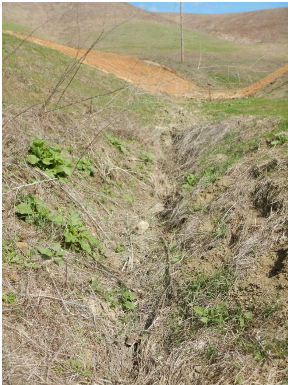
Figure 23. Downstream headcutting and erosion.
