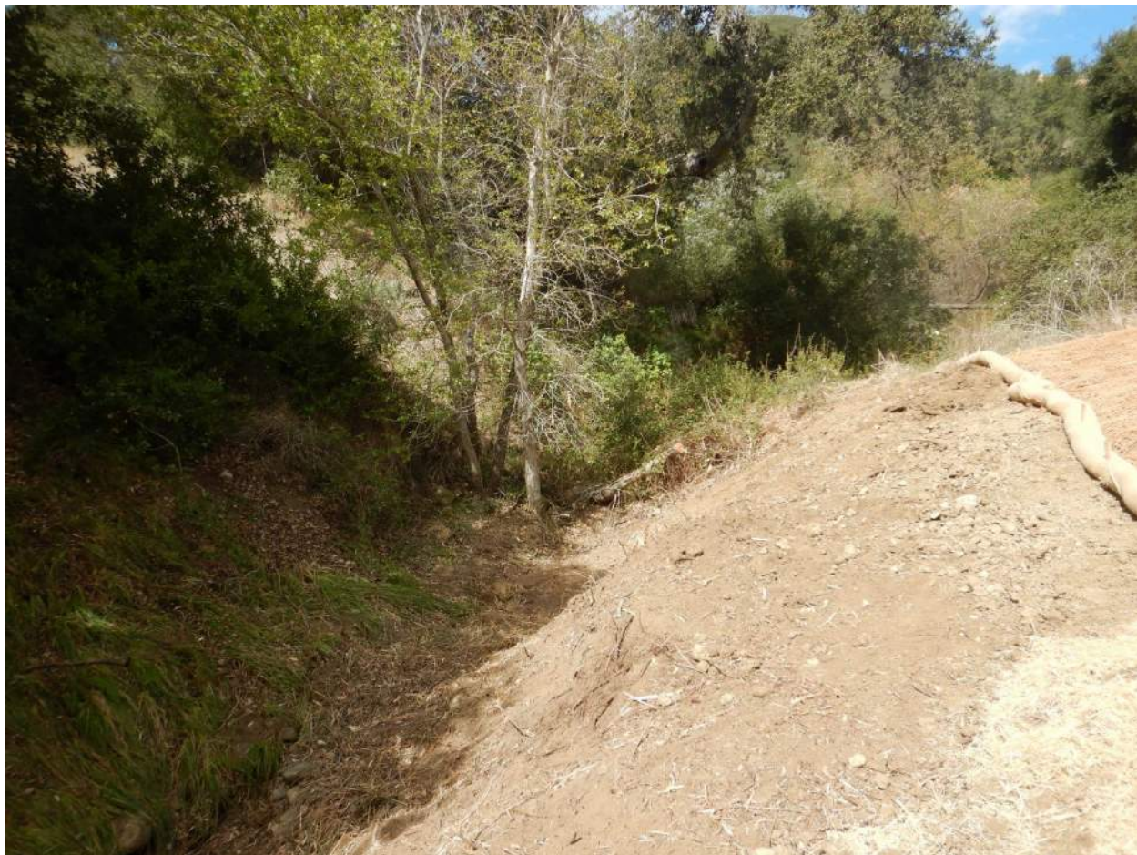
Figure 30. Cleared vegetation and loose sediment discharged to channel.
