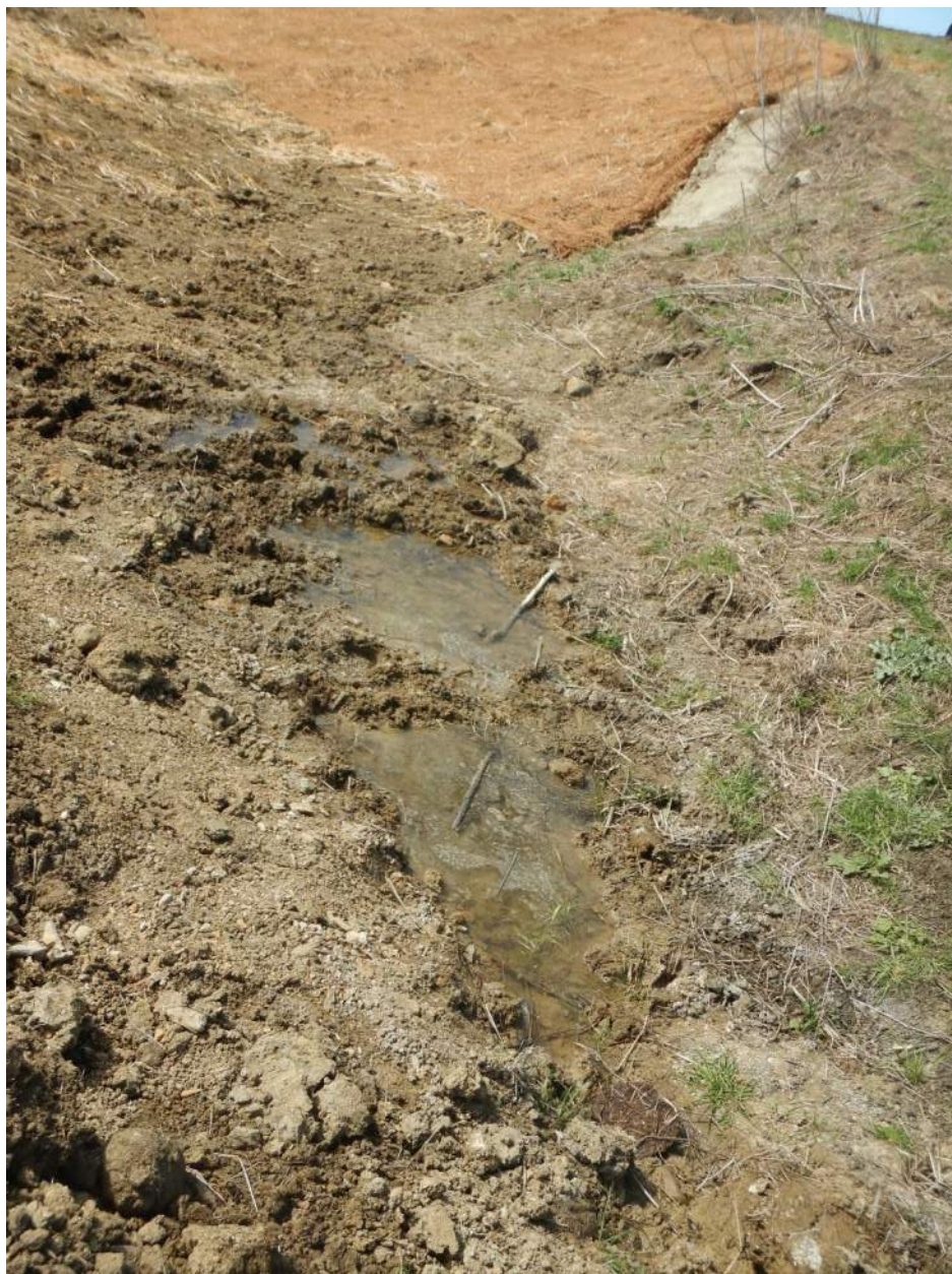
Figure 25. Example of pools of standing water seen in channel. Area of disturbance in channel is wetted and subject to erosion.
