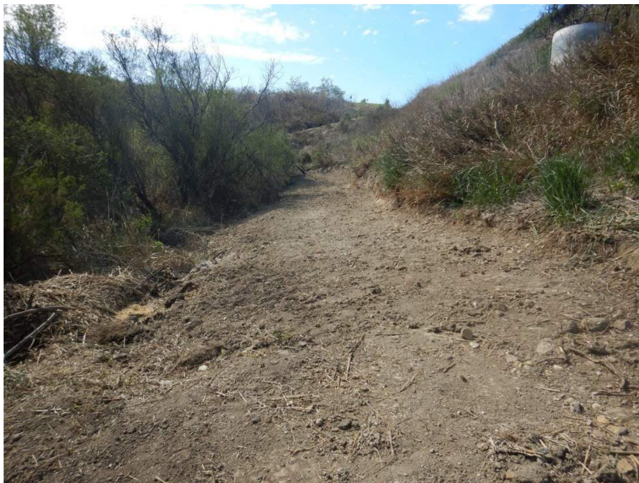
Figure 7a. Road grading without erosion control BMPs.
