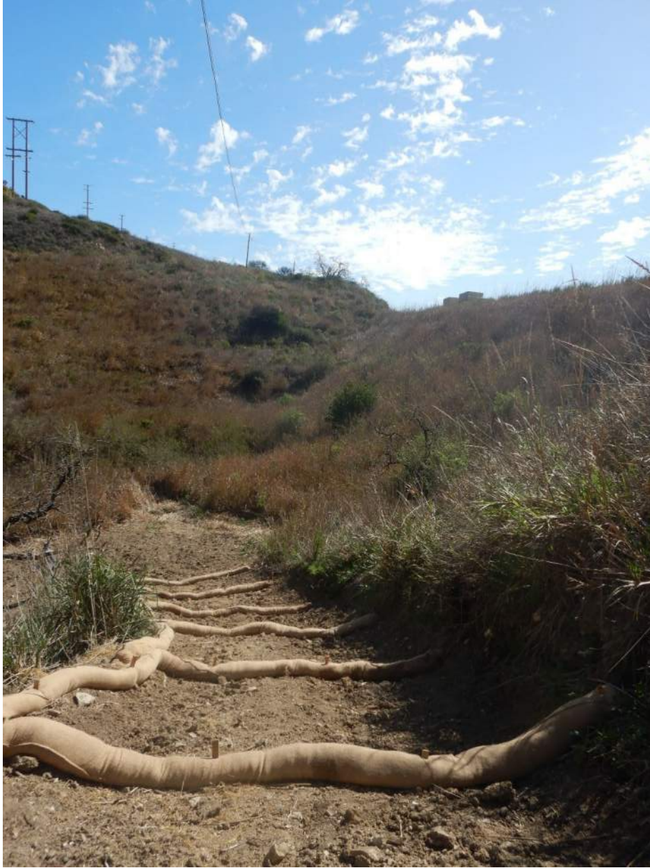
Figure 7b. Road to work site with BMPs installed. This is the road that heavy equipment would have traversed to access the worksite.
