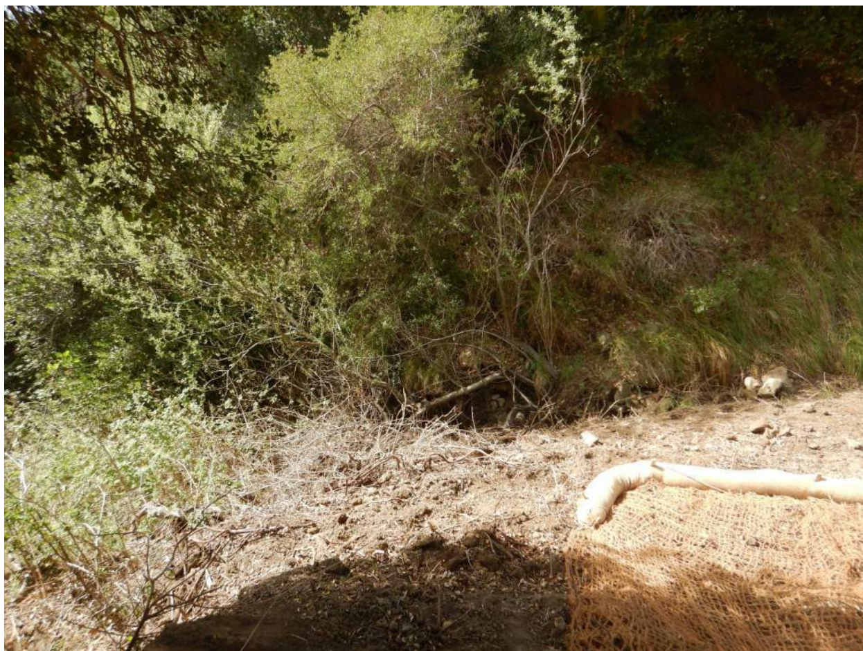
Figure 29. Work site extends beyond TOB. Loose sediment and vegetative debris are inadequately secured.
