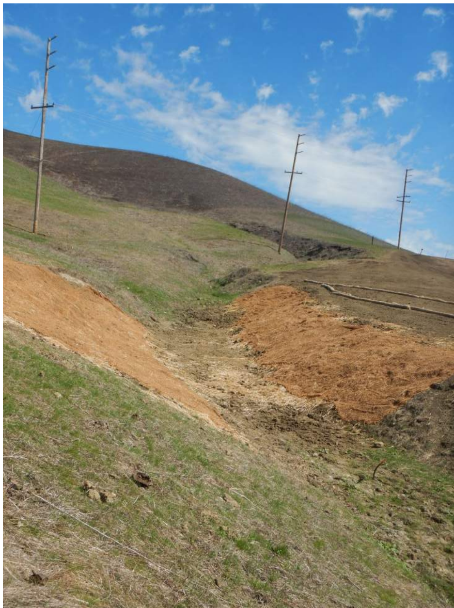
Figure 22. View of work site. Disturbed soils in channel, vegetation removed from banks and upland staging area, dry vegetation discharged to channel.
