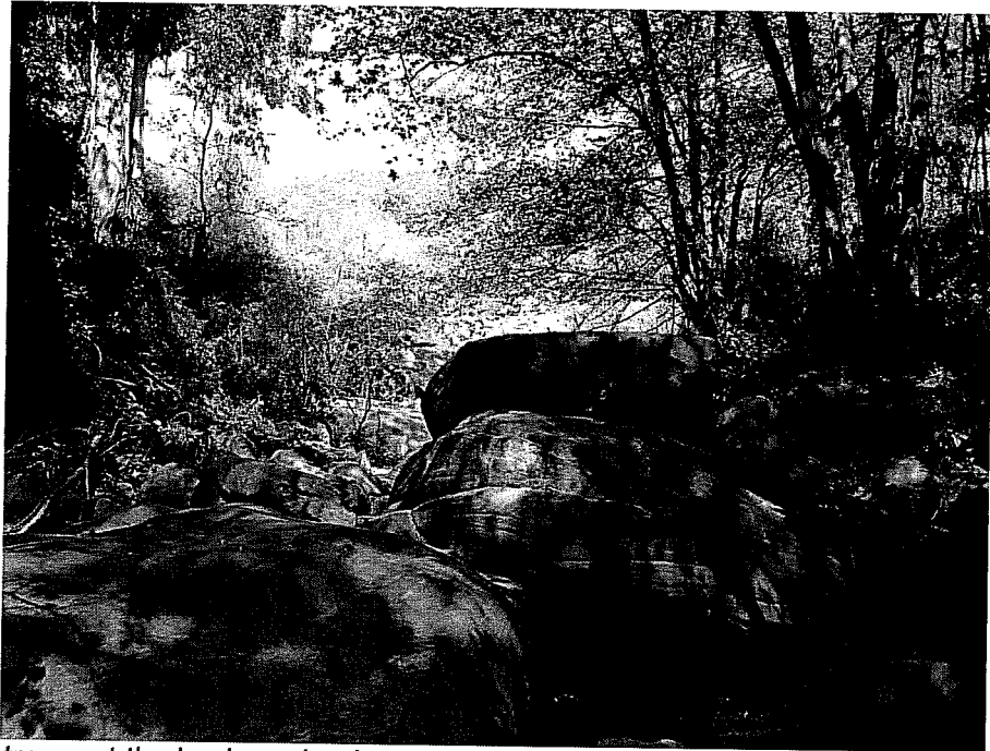
Looking upstream at the basin embankment showing impassable boulders. The access road transitions from the creek invert up onto the east bank approximately 75 feet downstream of these boulders.
