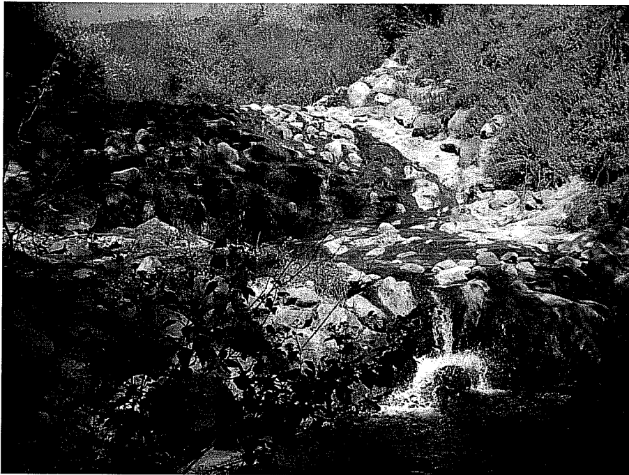
Looking upstream at the basin embankment
