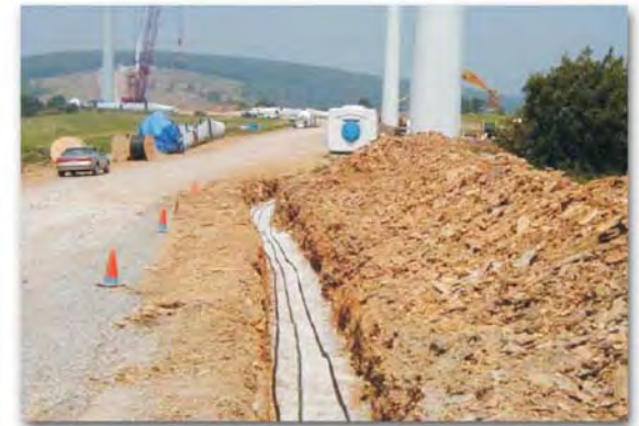
Inset C: Excavated trench for underground cables.
