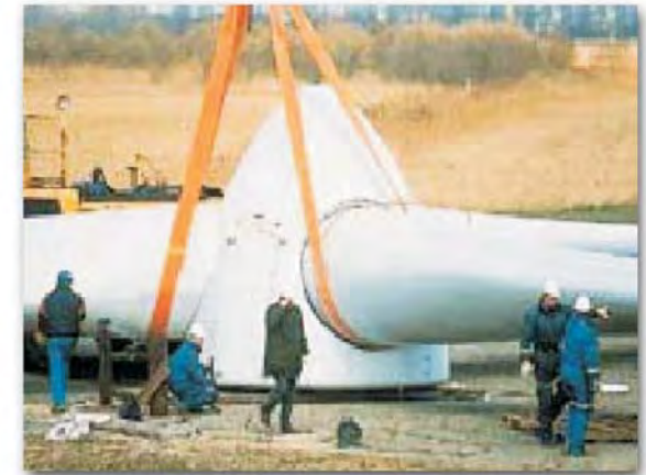
Inset F: WTG blade/hub assembly.
