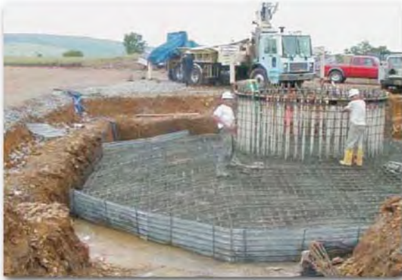
Inset A: WTG Foundation construction.
