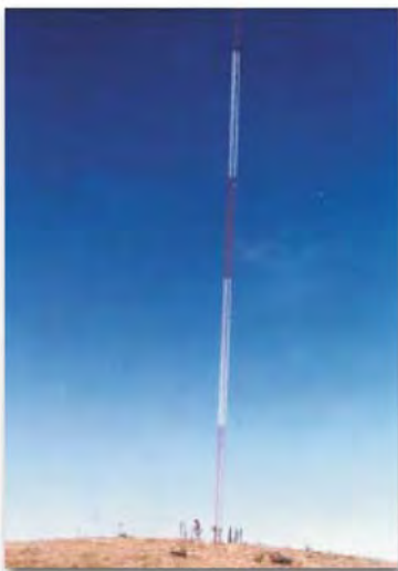
Inset G: Meteorological tower.
