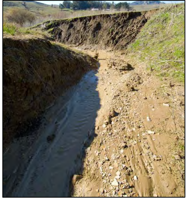
PHOTO 2 Looking South from Blue-line Feature Crossing 2
