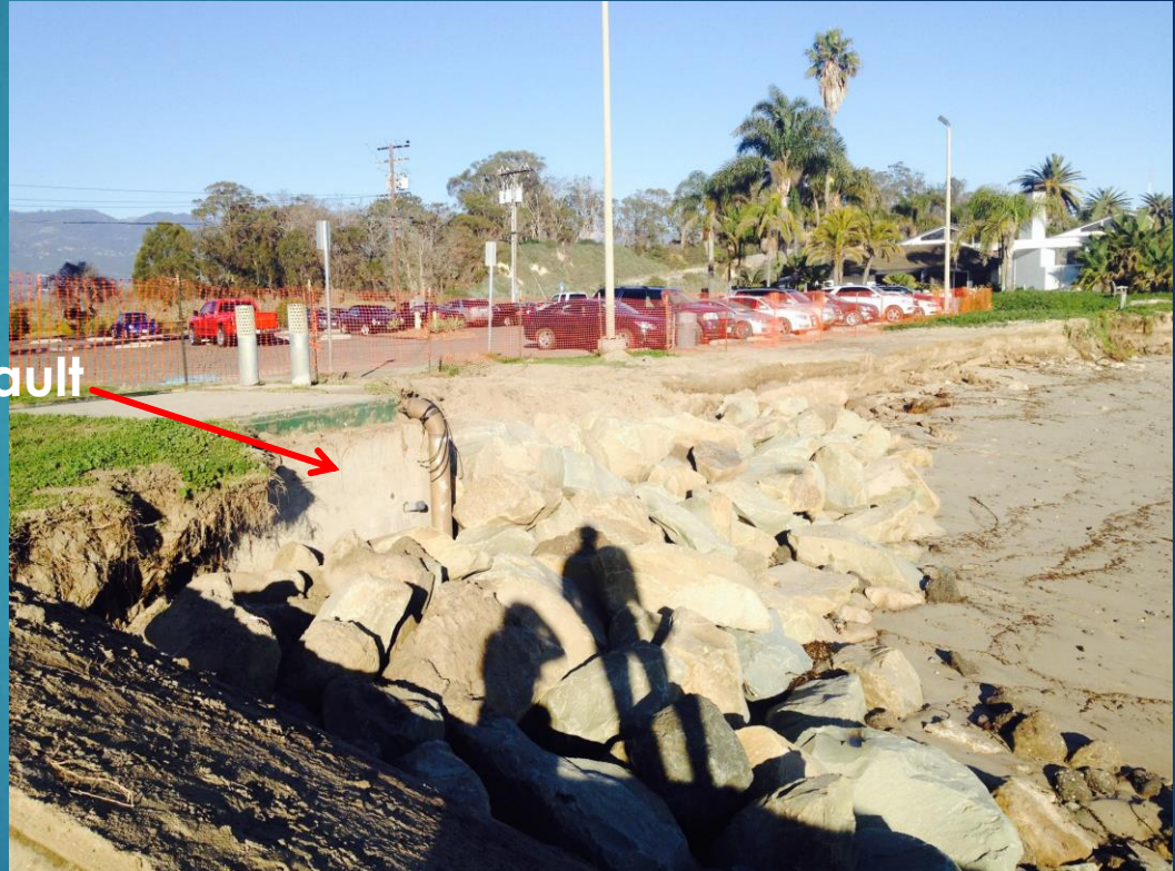
Rock protection for Goleta Sanitary sewer outfall vault installed by GSD
