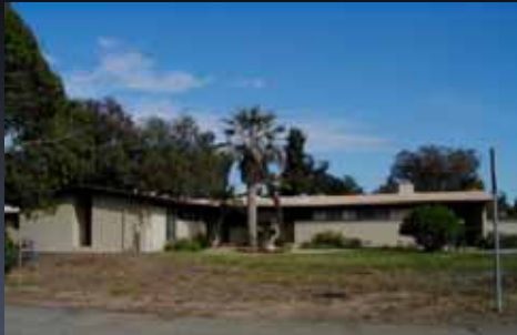
Projected Completion March 2006
