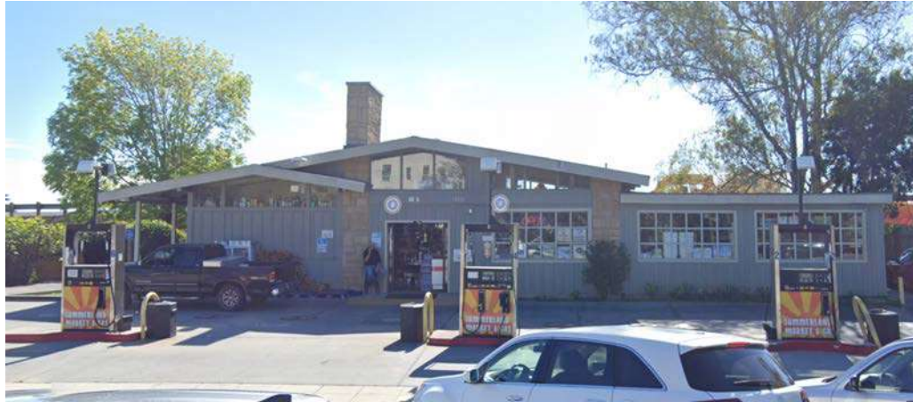
1. Front view of existing gas station
