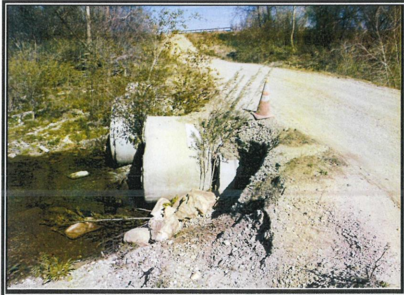
Looking North at Arizona Crossing (#788)
