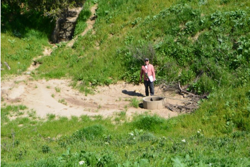
Photo 31. Crossing #3: 32-in. RCP culvert inlet structure that conveys water from man-made drainage system (Class IV watercourse) underneath gravel access road and gravel pad. (photo taken 3/26/2019)
