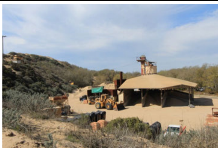
The Gordon Sand Company is a commercial sand mining operation that includes a sand screening and processing facility as well as an access road and sand collection pits. Access to the site is provided by a remnant unpaved road.
