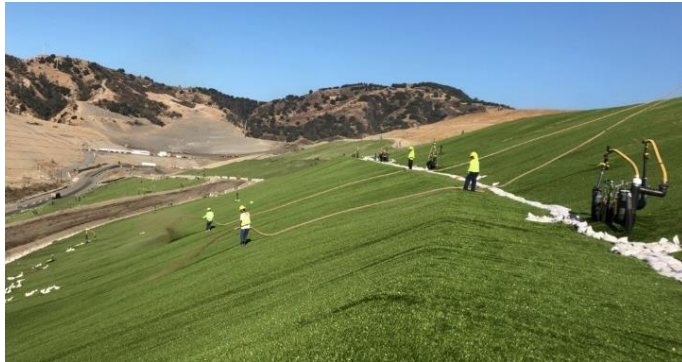
Installation crew spraying infill sand into the newly installed closure turf.
