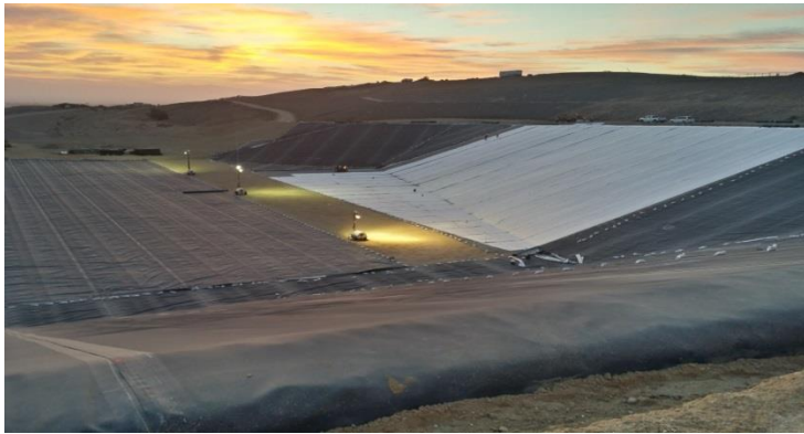
CQA during liner installation at Taft Landfill.
