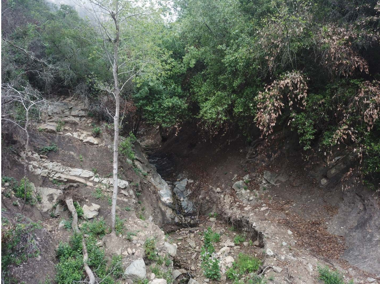
Site BV-6 Photo by Kane Geotech (2018.05.29)
