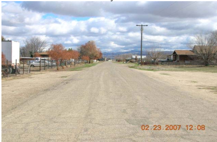
Before - Johnson Street in Cuyama
