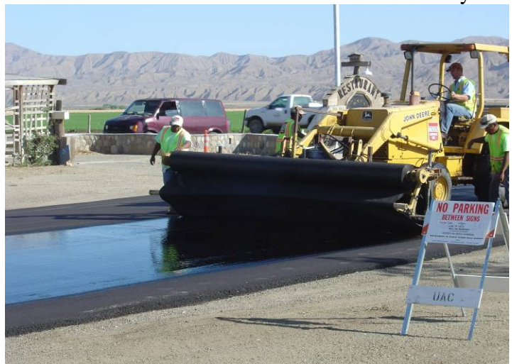
Construction in Cuyama
