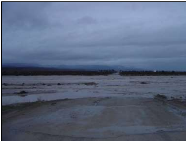
Existing Foothill Road Low Water Crossing over the Cuyama River, looking westerly
