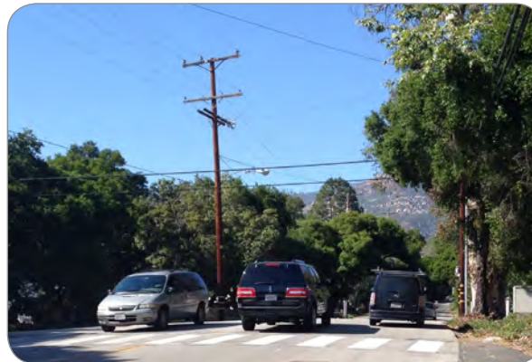
POWER LINES AND STREET LIGHTS
