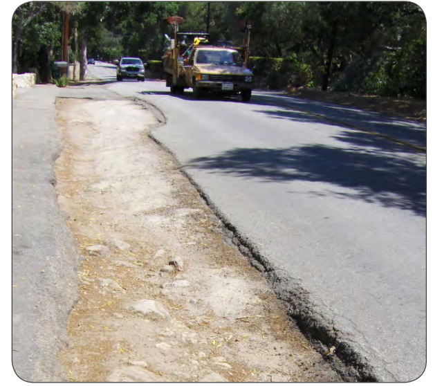
WALKWAY AND DRAINAGE ALONG MISSION CANYON ROAD
