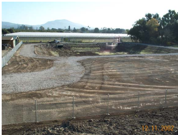
Franciscan Sediment Basin Project Completion
