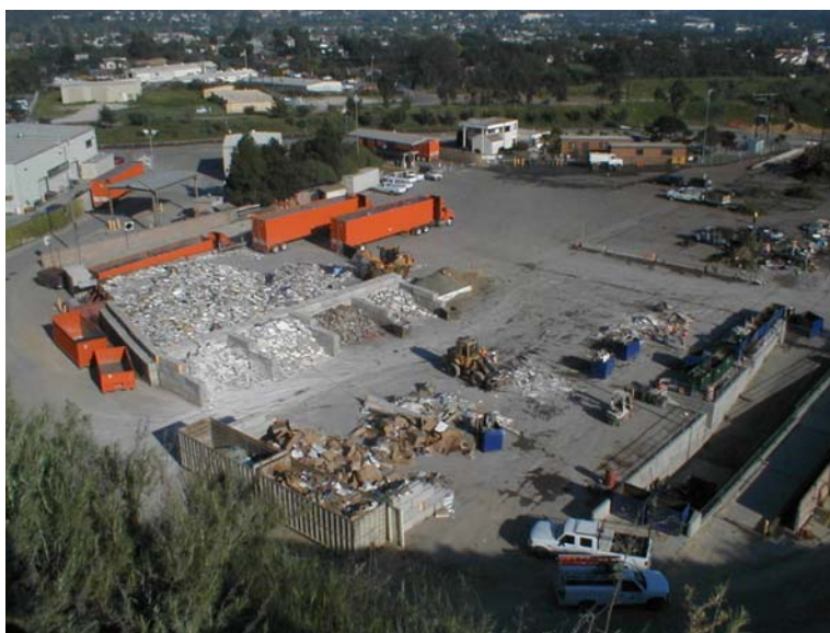
South Coast Transfer Station C&D Sorting Area
