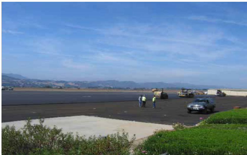
Photo: Current Apron Construction at Santa Ynez Valley Airport
