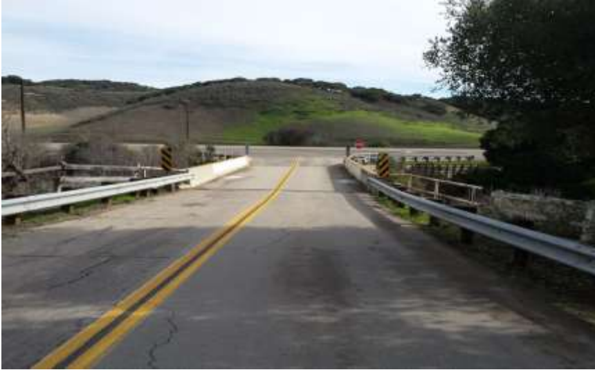
Jalama Road looking east at State Route 1, May 2016
