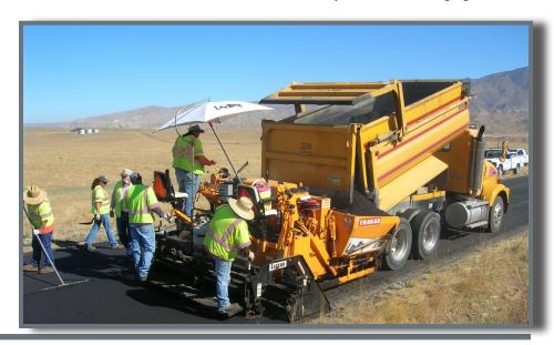
perform in-house leveling maintenance operations to correct failed and distressed areas in the roadway. In many cases, staff can repair the roadway and bring it to an acceptable standard using an asphalt leveling course. This consists of a thin layer of either cold or hot asphalt applied to the entire pavement width, covering the failed areas of the roadway. Essentially, the in-house leveling operation is a large patch that strengthens pavement distress and improves ride-ability.
