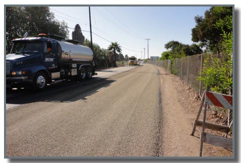
gallon per square yard. This seals the asphalt and prevents fines loss and water from penetrating the roadway thereby extending the life of the pavement by one to two years. Maintenance forces perform fog sealing as a maintenance activity.
