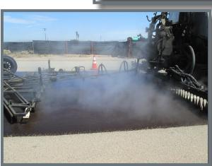
3. An even coat of chips or other readily available aggregate is applied over the emulsion.
