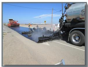
2. A specially designed drag broom is then pulled through the emulsion to fill cracks and voids left open by the initial application.
