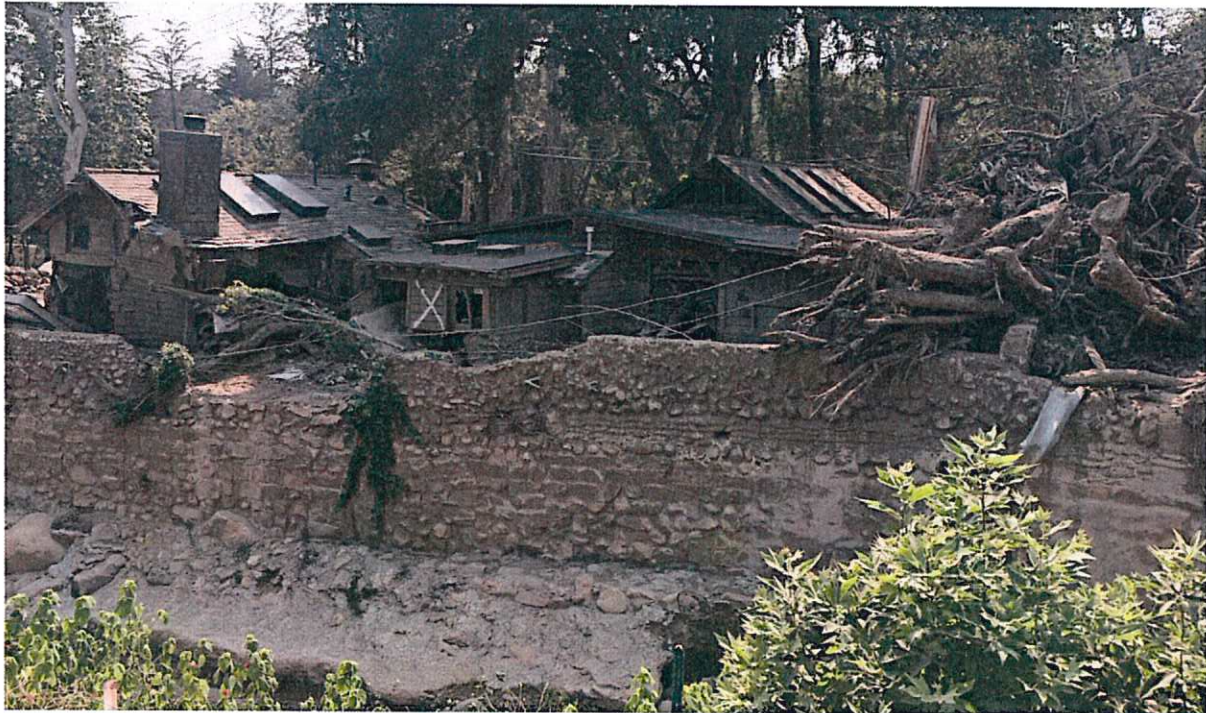
Figure 10. Woody debris immediately upstream of a destroyed home on Montecito Creek located approximately 2 km from the fan apex. BGC photo, July 2018, looking west.
