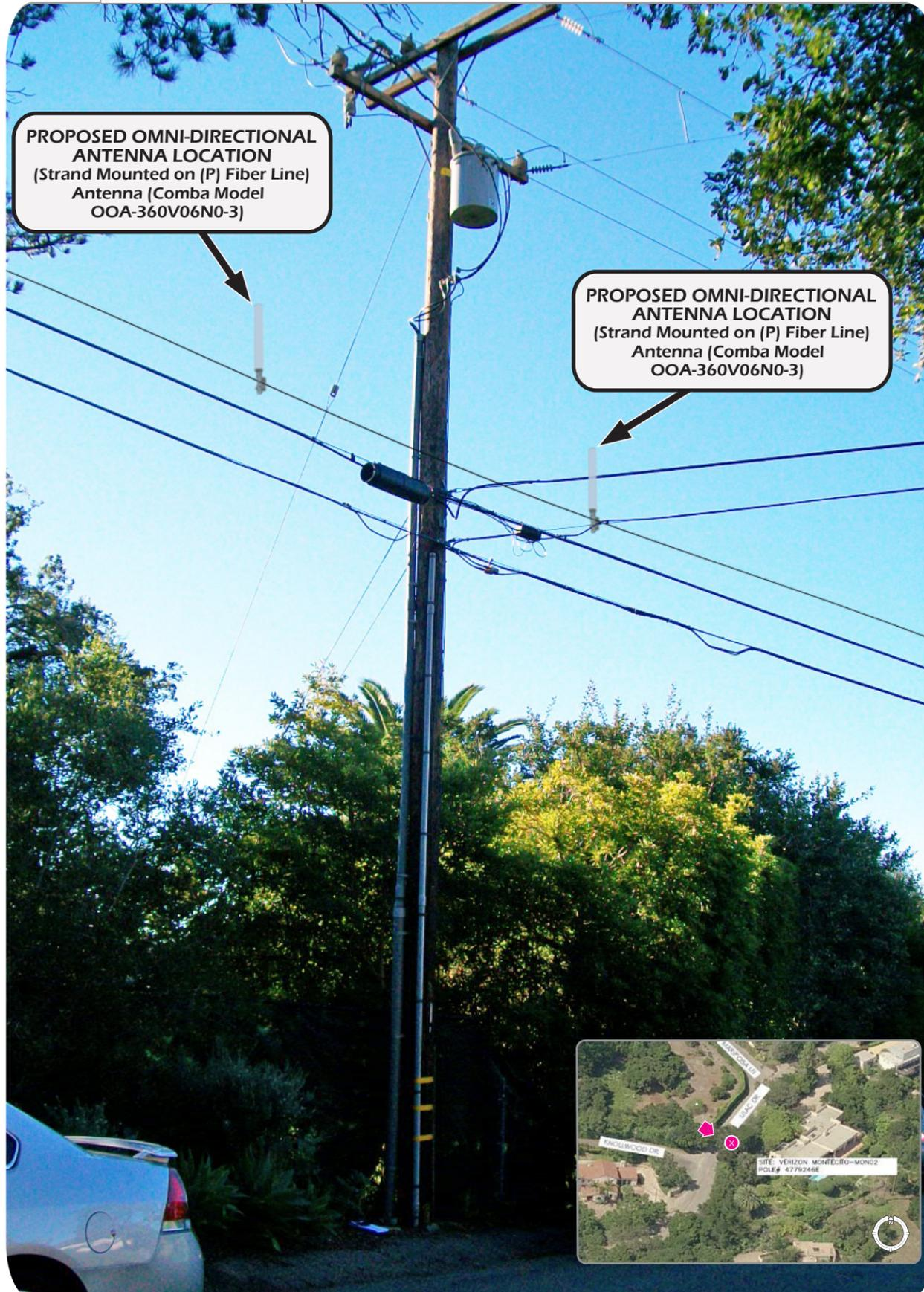
PROPOSED OMNI-DIRECTIONAL ANTENNA LOCATION (Strand Mounted on (P) Fiber Line) Antenna (Comba Model OOA-360V06N0-3)
