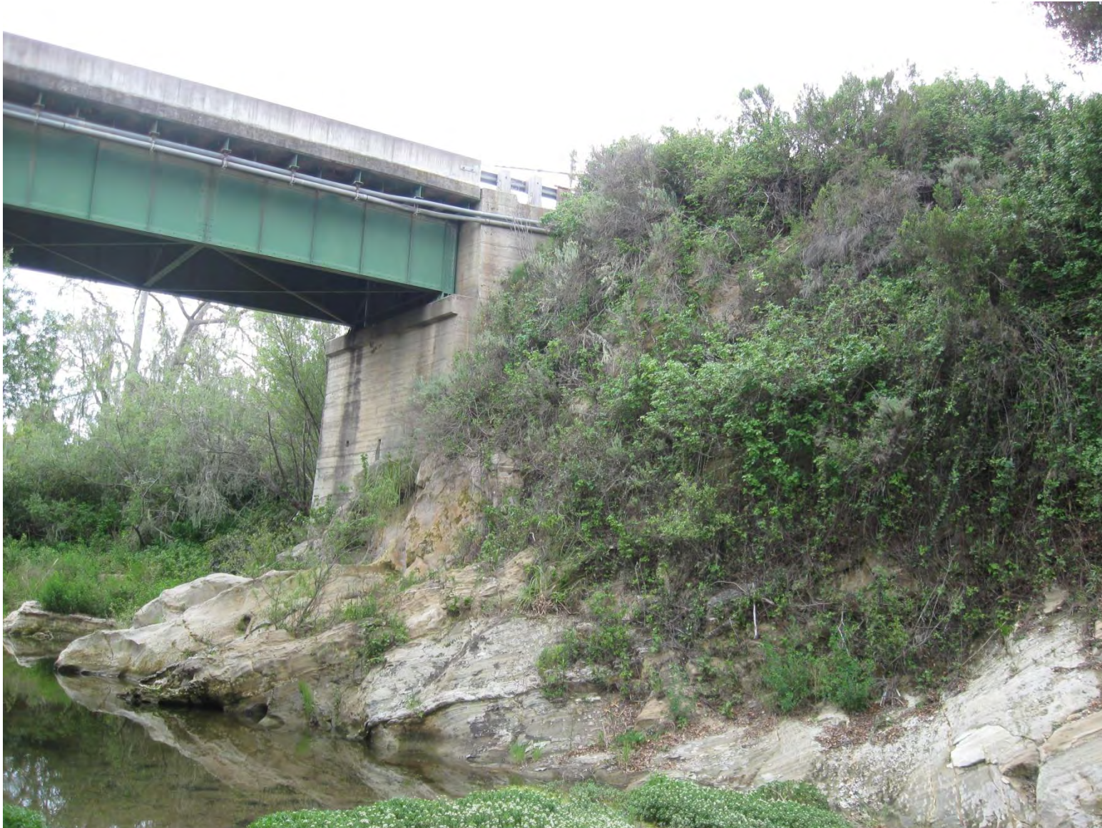
Photo 11 Looking at northwest slope
