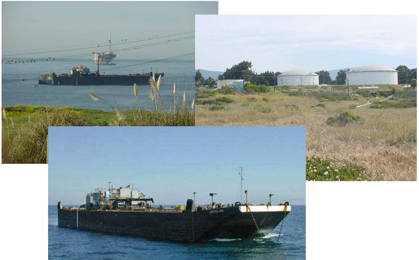
Figure 8: Upper left: view of Platform Holly and Barge Jovalan from shore. Upper right: two 65,000-barrel crude oil storage tanks and 10,000-barrel firewater tank. Lower center: single-hulled Barge Jovalan.
