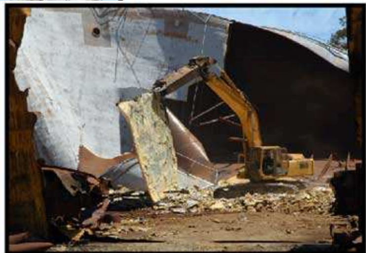
Figure 13: Former Gaviota Marine Terminal
