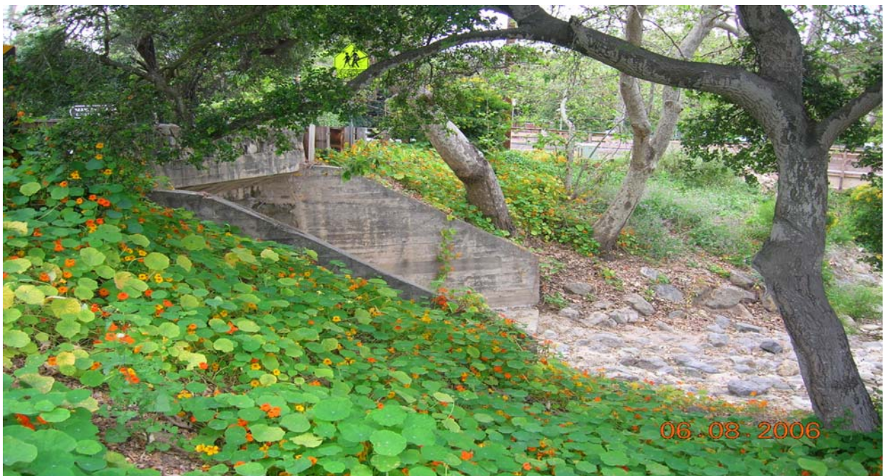
View east, proposed project location
