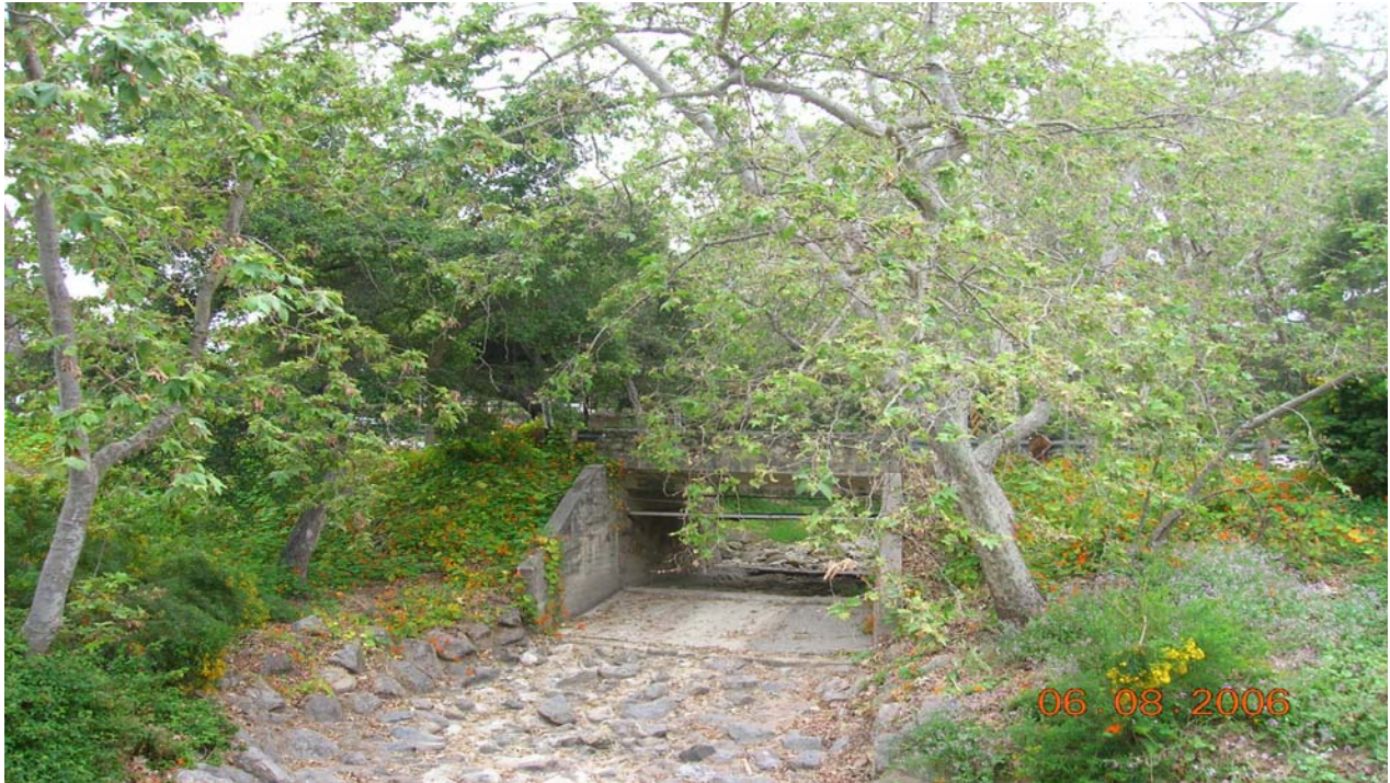
View north, Santa Rosa road bridge 51C-045 over Oak Creek.
