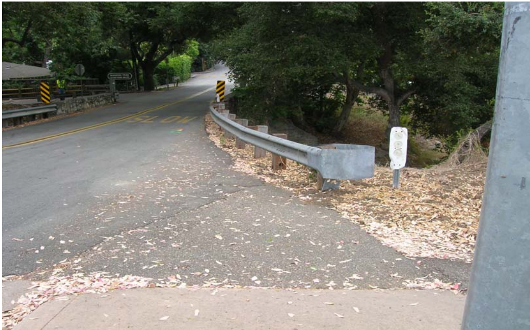
Photo: Existing Santa Rosa Lane Bridge (No. 51C-045) over Oak Creek looking east along proposed pedestrian bridge alignment.
