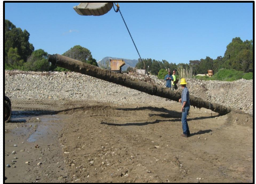
Pipeline being removed April 19, 2011
