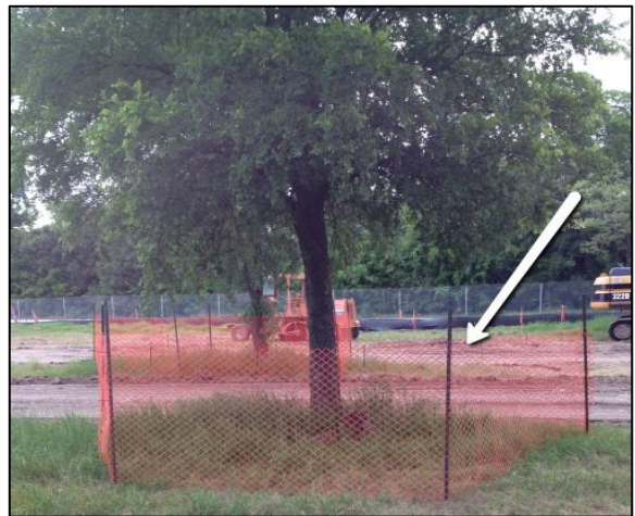
Orange Mesh Temporary Fencing Example 3
