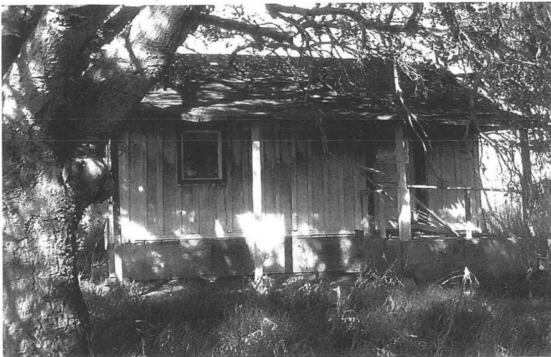
Staff Cottage, south elevation, looking north.
