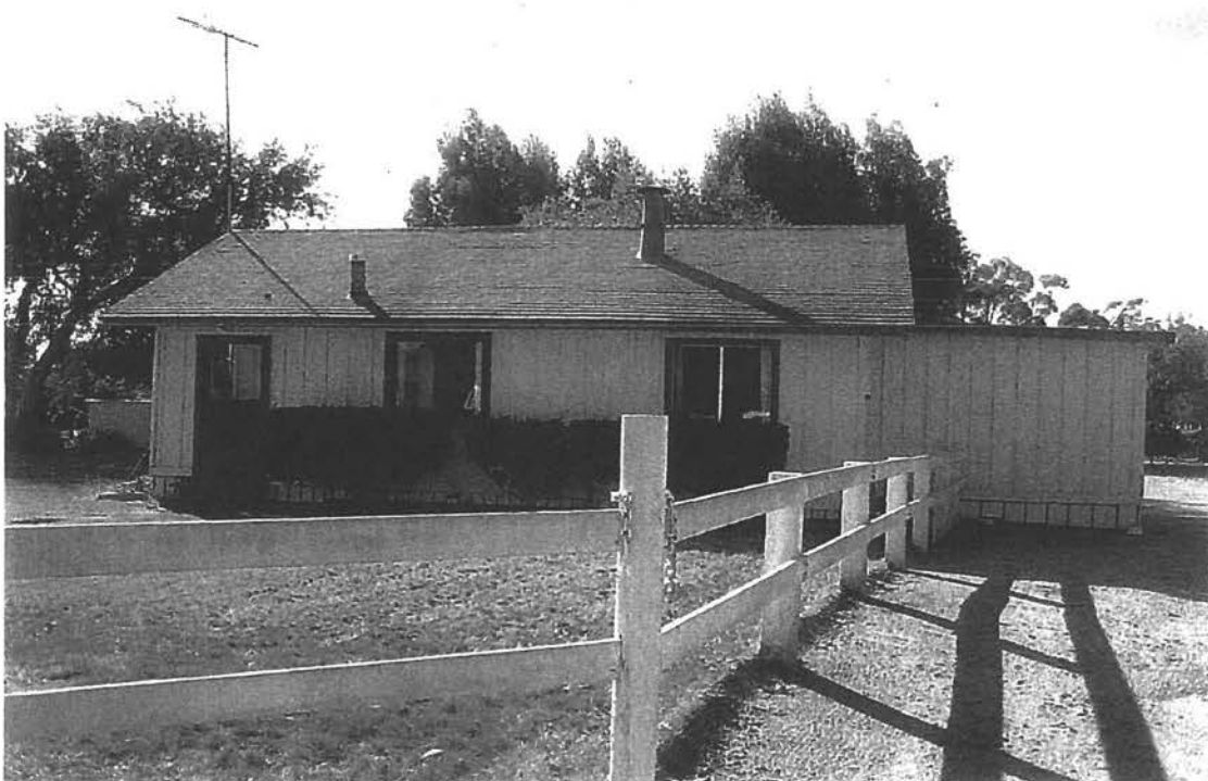
Staff Cottage No. 1, east elevation, looking west.
