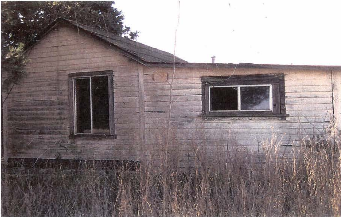
Staff Cottage, partial east elevation, looking west.
