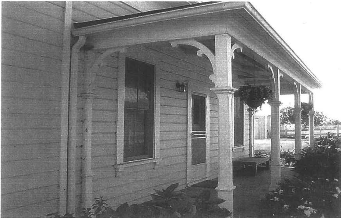
Main House, porch detail, north elevation, looking southwest.
