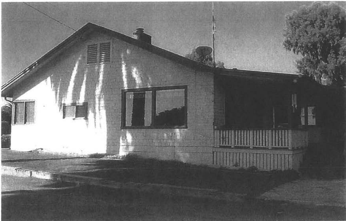
Foreman's House, south elevation, looking northwest.
