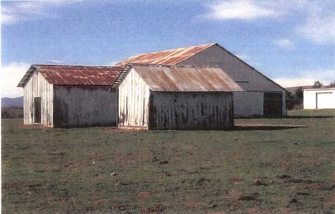
From foreground, Barn Nos. 3, 2, 1, looking northwest.
