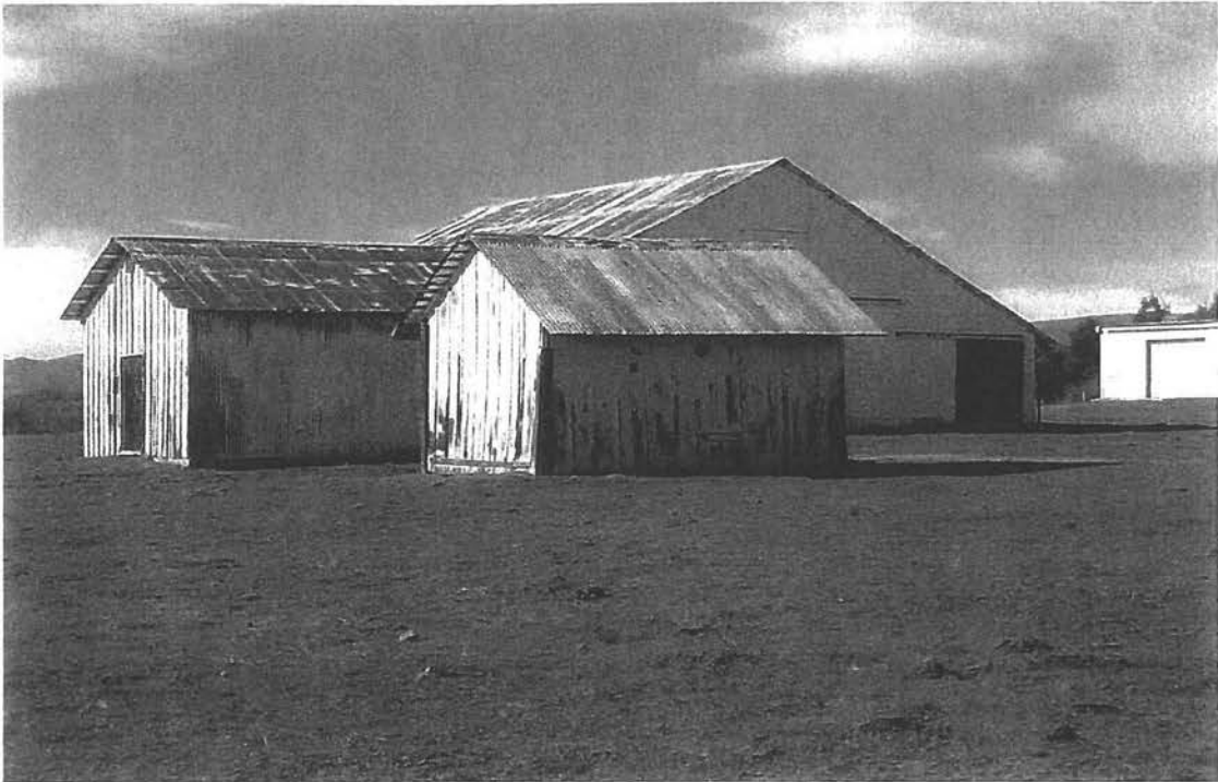
From foreground, Barn Nos. 3, 2, 1, looking northwest.
