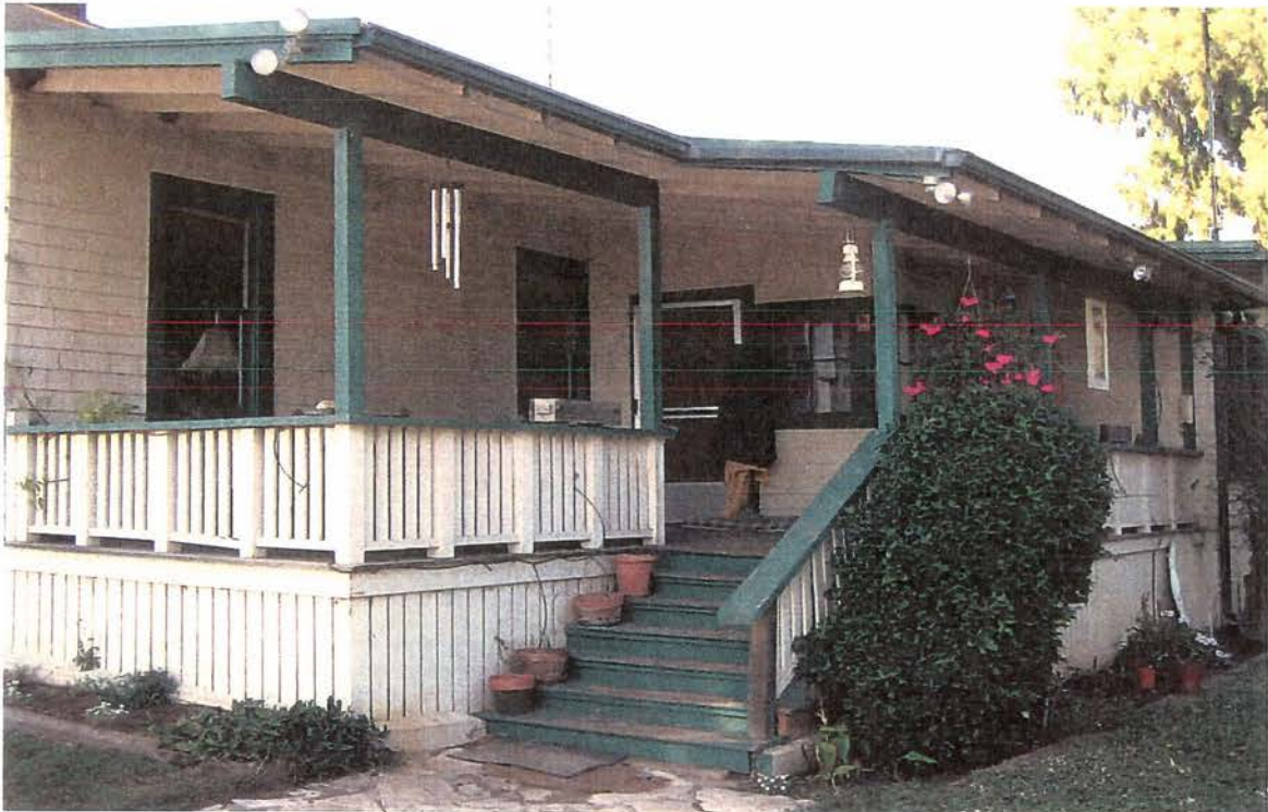
Foreman's House, partial east elevation, looking northwest.
