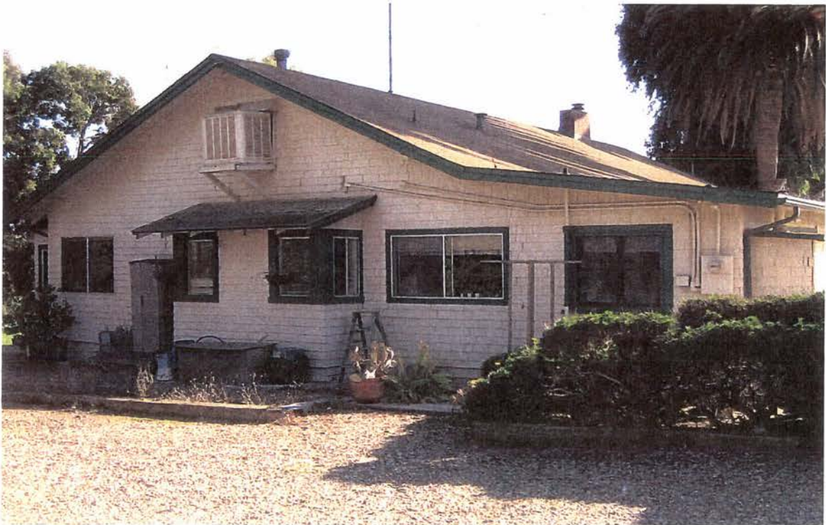
Foreman's House, north elevation, looking southeast.
