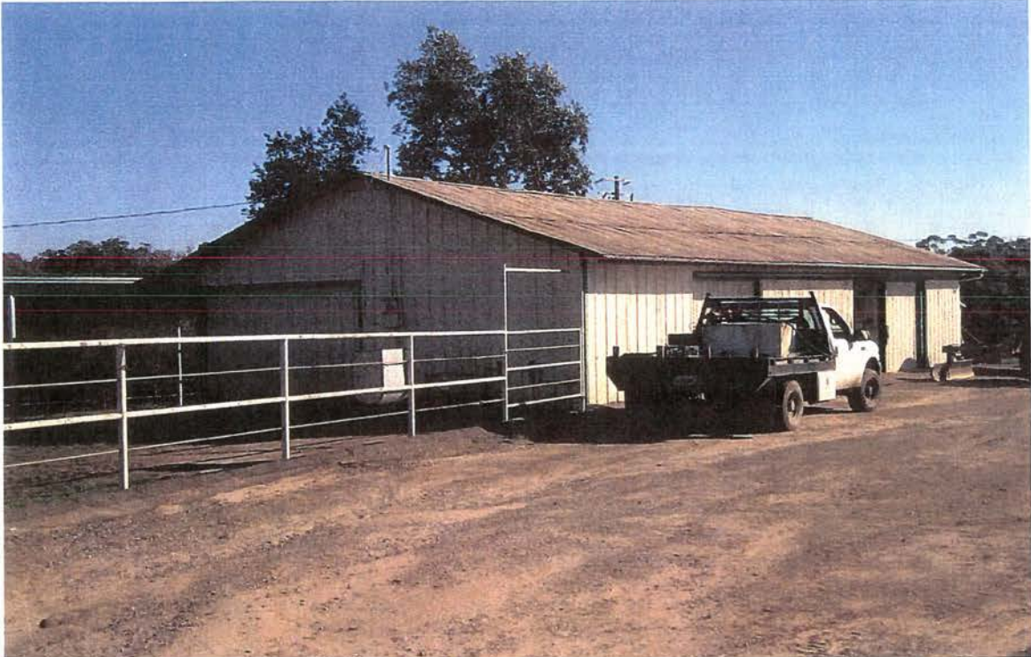
Repair Garage, north and west elevations, looking southeast.
