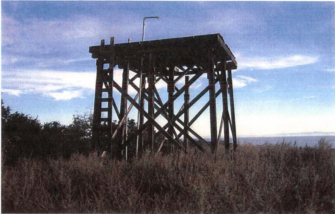
Water Tank Tower, north elevation, looking southeast.
