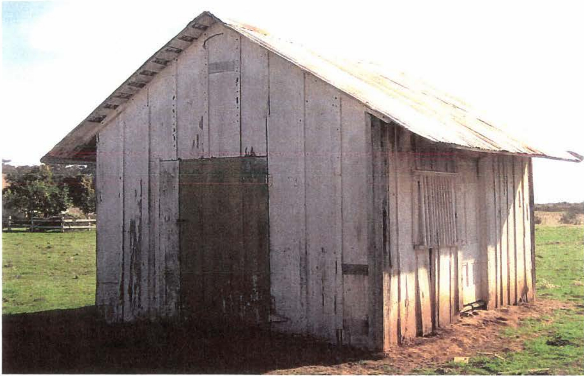
Barn No. 3, north and west elevations, looking southeast.
