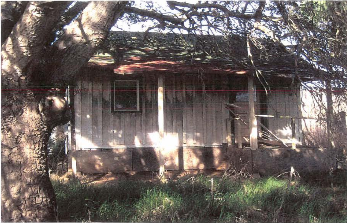
Staff Cottage, south elevation, looking north.
