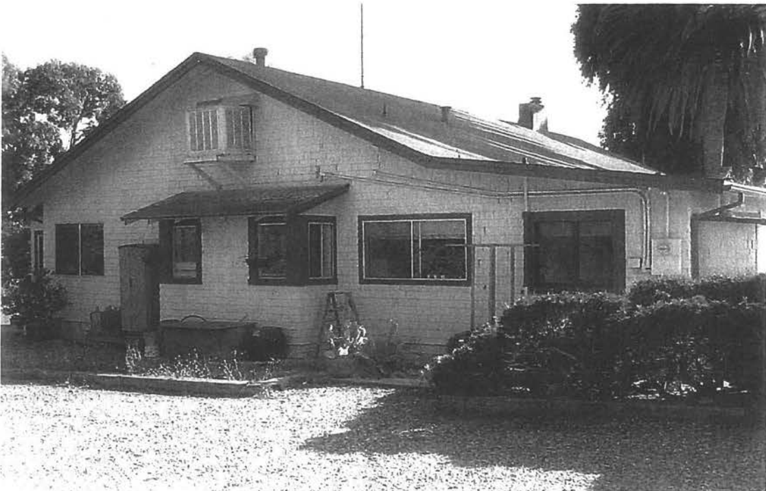
Foreman's House, north elevation, looking southeast.
