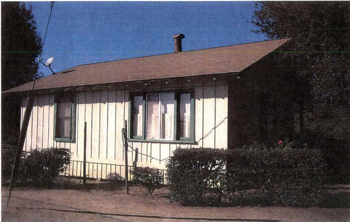
Staff Cottage No. 2, south and east elevations, looking northwest.
