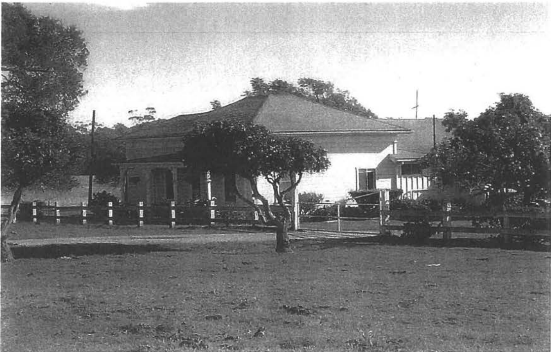
Main House, north and west elevations, and landscape, looking southeast.
