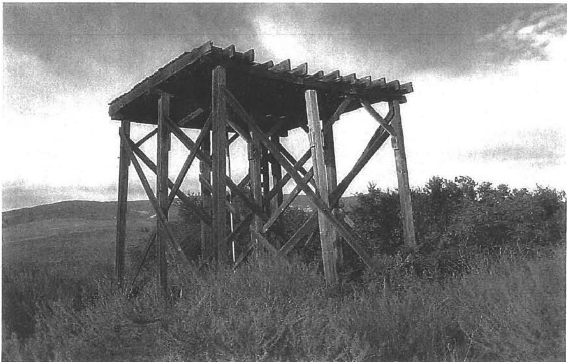
Water Tank Tower, west and south elevations, looking northeast.
