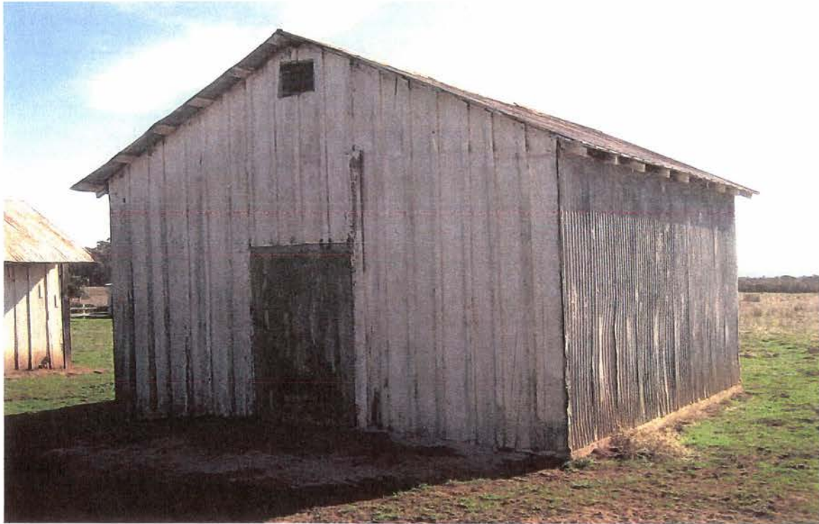
Barn No. 2, north and west elevations, looking southeast.
