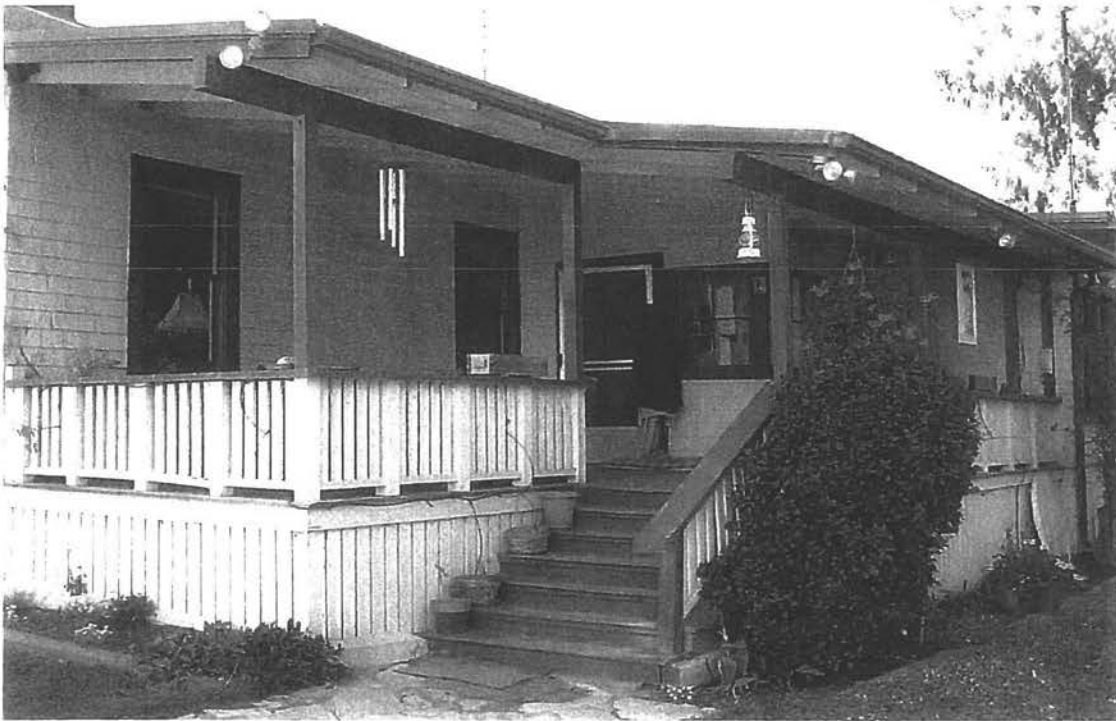
Foreman's House, partial east elevation, looking northwest.
