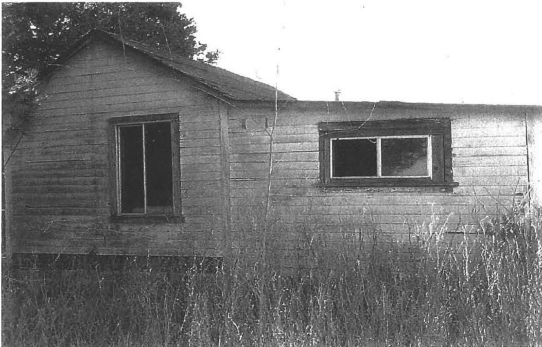
Staff Cottage, partial east elevation, looking west.
