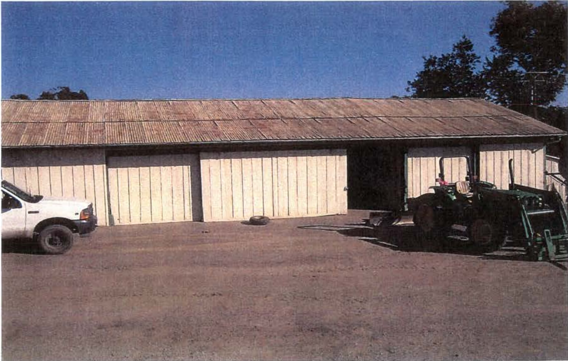
Repair Garage, west elevation, looking east.
