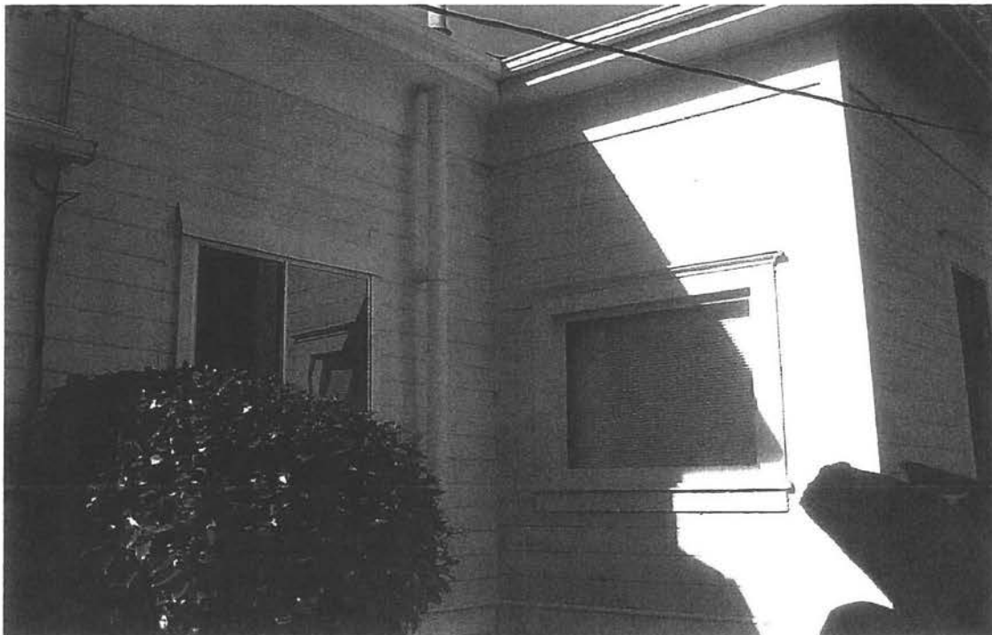
Main House, window detail, east and south elevations, looking northwest.
