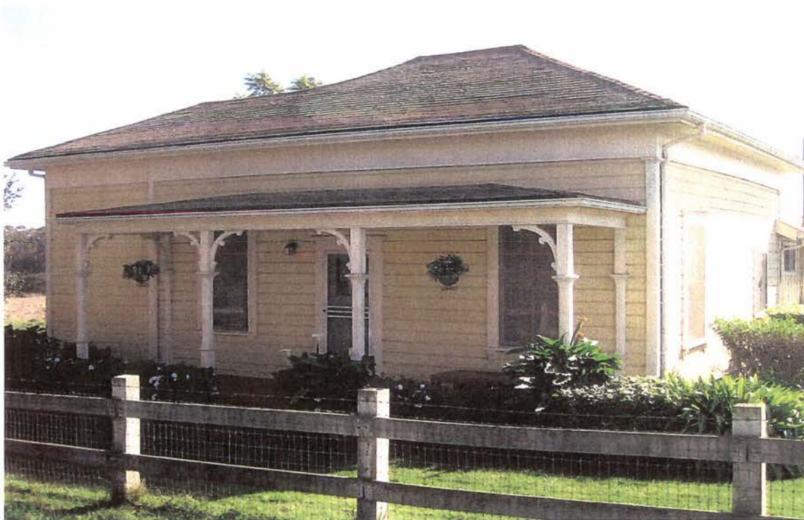
Main House, north elevation, looking southeast.
