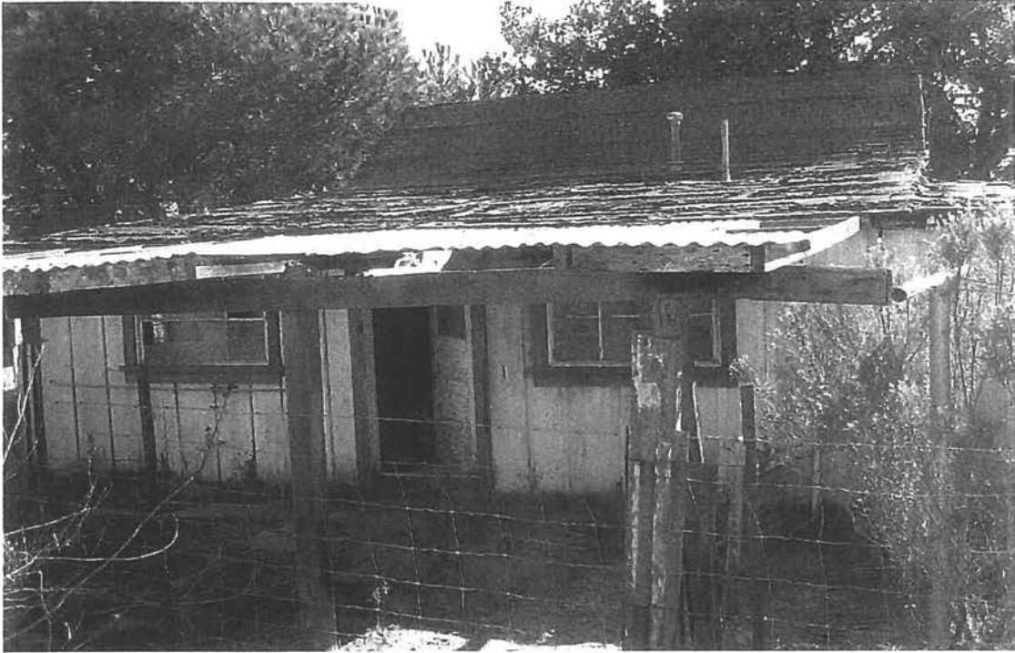
Staff Cottage, north elevation, looking southeast.
