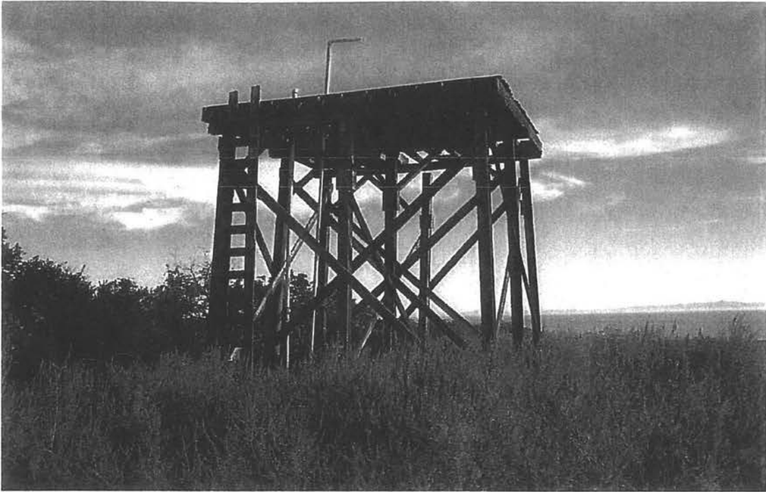
Water Tank Tower, north elevation, looking southeast.
