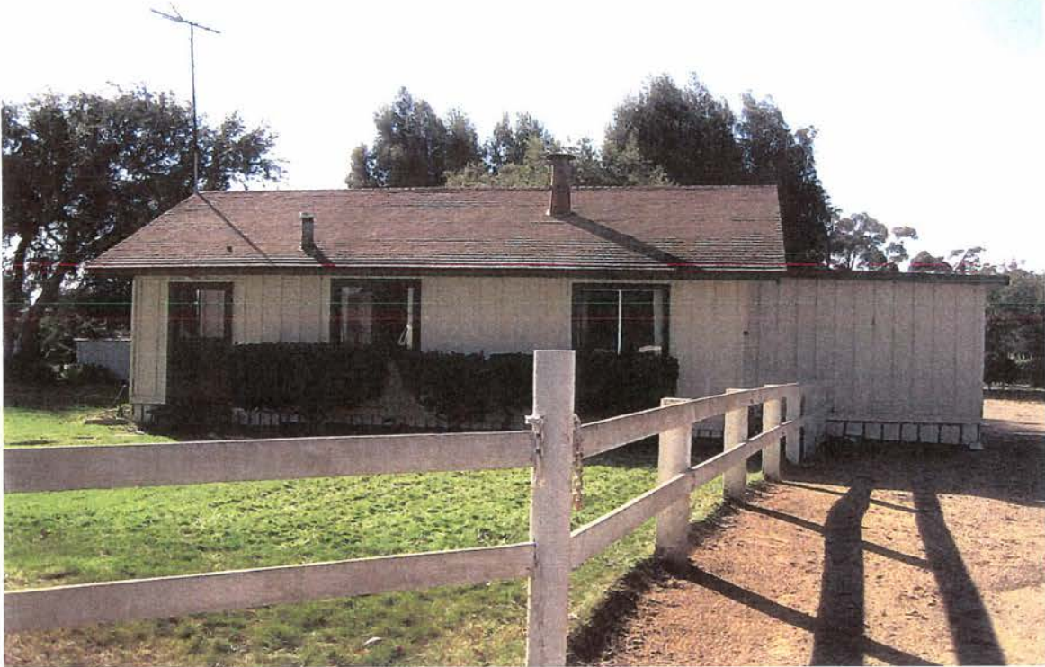
Staff Cottage No. 1, east elevation, looking west.
