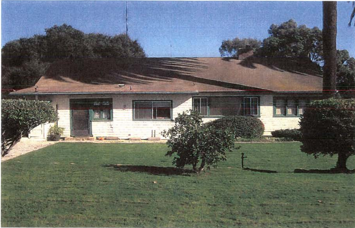
Foreman's House, west elevation, looking east.
