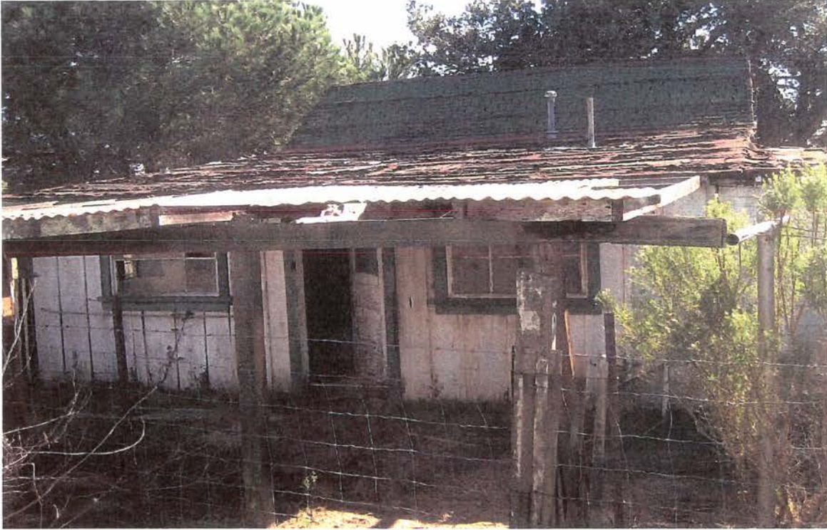
Staff Cottage, north elevation, looking southeast.
