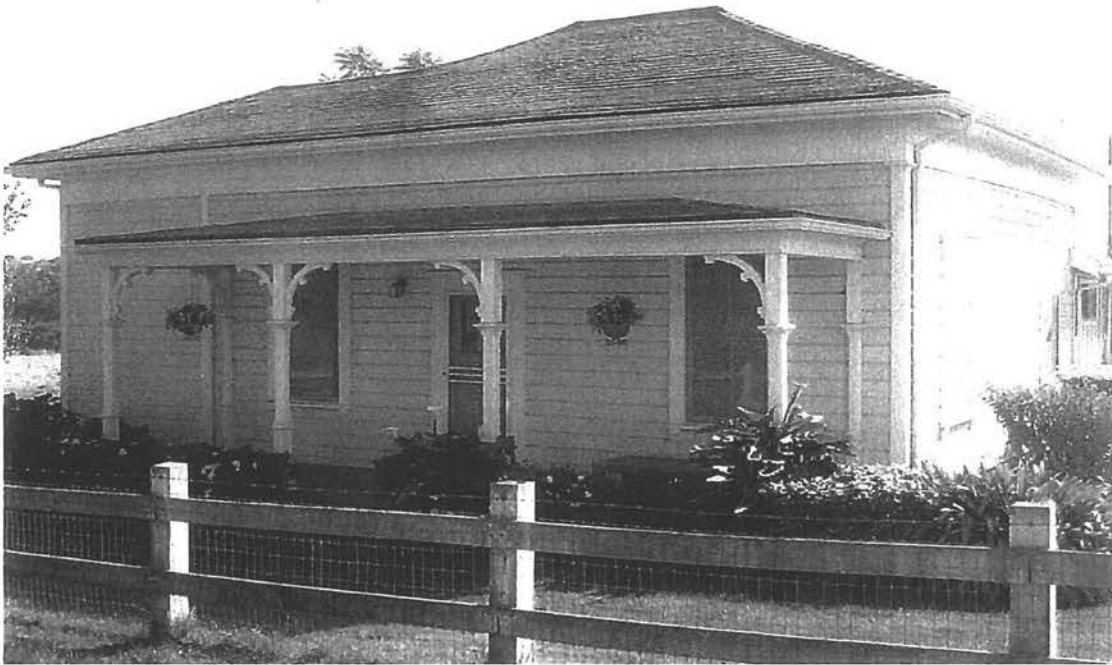
Main House, north elevation, looking southeast.
