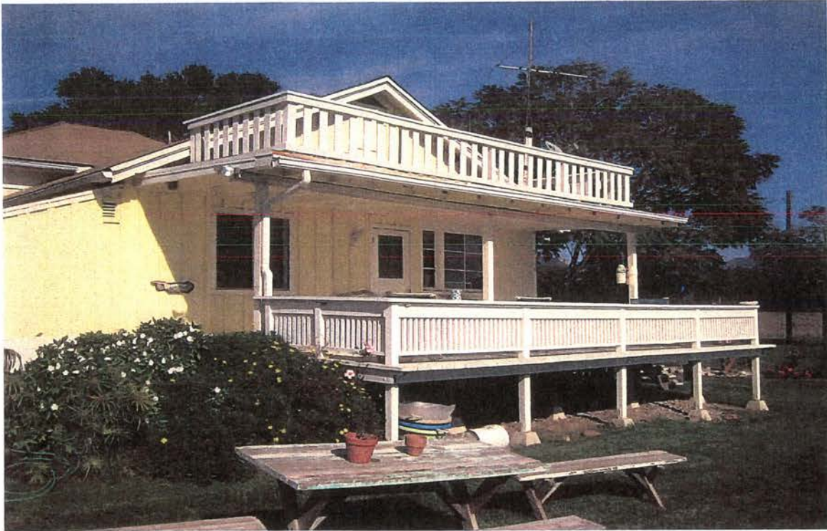
Main House, south elevation, looking northeast.
