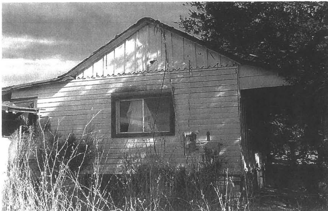
Staff Cottage, partial west elevation, looking east.
