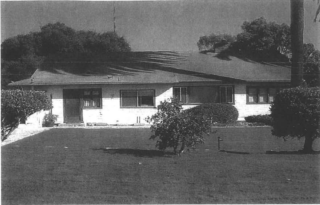
Foreman's House, west elevation, looking east.
