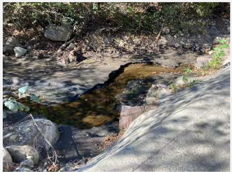
Soil deposited in Refugio Creek following the 2021 Alisal Fire.
