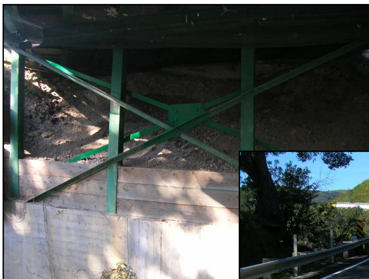
Jalama Road Bridge at Ramajal Creek- No. 51C-016
