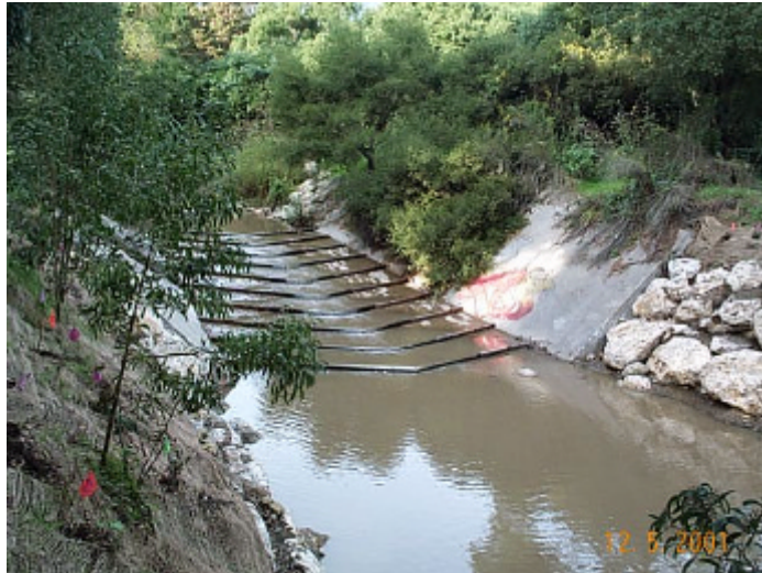
Completed Check Structure Modification
