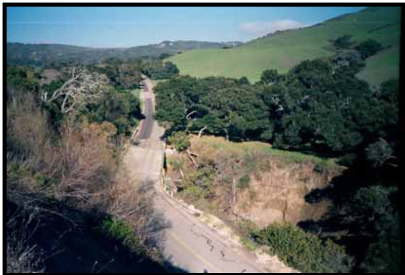
Photo: Existing Jalama Road embankment and roadway conditions
