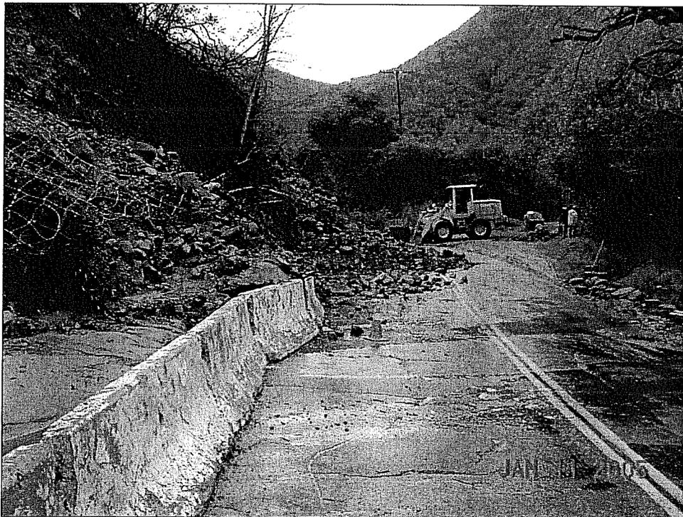
**Stagecoach Road, with existing netting showing contained materials and adjacent, unprotected area where rock debris entered the roadway.**
