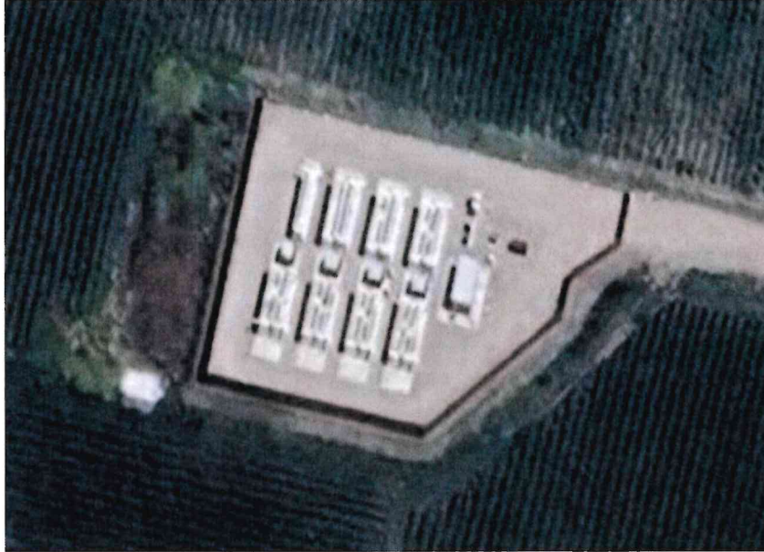
Vallecito Energy Storage Resilience Project. Tesla Battery Energy Storage System, 10 MW and 40 MWh, located on 1 acre of land in Carpinteria near the electrical substation (operational since 2021)
