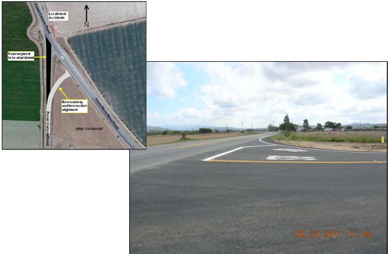
Completed Intersection at Foxen Canyon Road and Santa Maria Mesa Road
