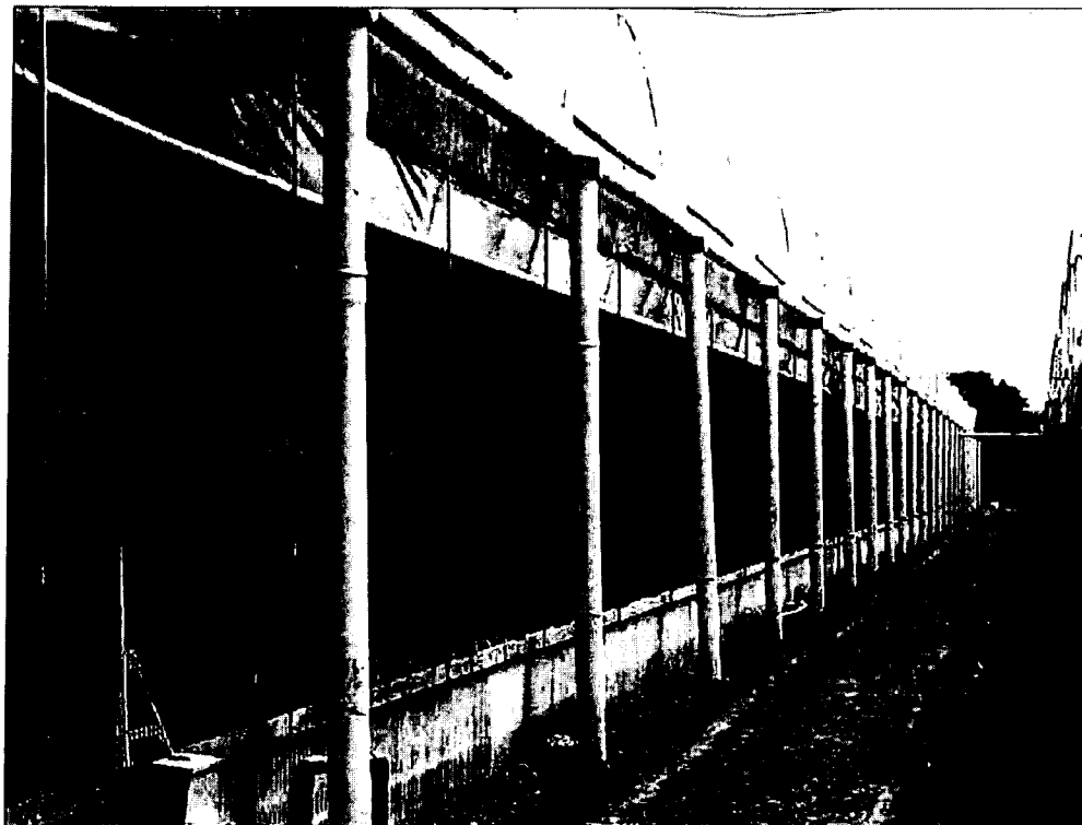
The above open-sided greenhouses located at 1296 Cravens Lane are currently being used to cultivate cannabis under the County's Article X provisions and a State Provisional license.
