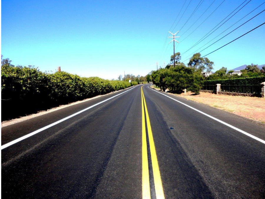
Areas showing Scrub Seal Process
