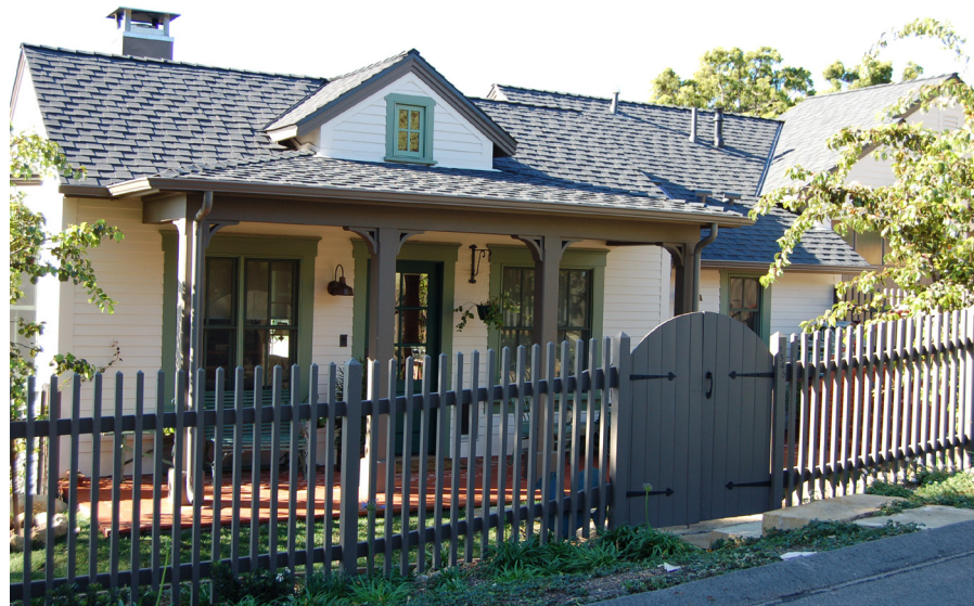
Figure 5.6 – Visible Front Entry with Defining Architectural Elements
