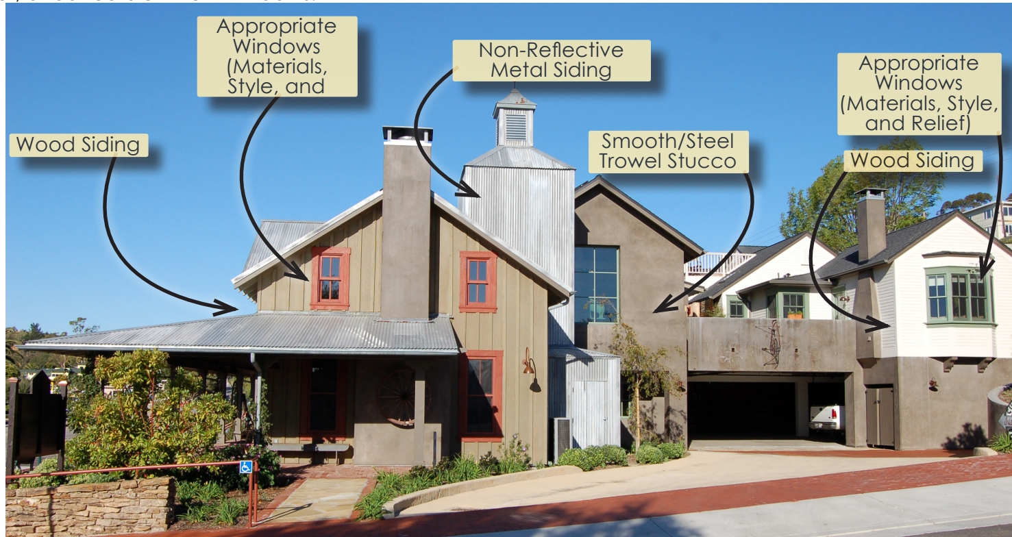
Figure 6.2 – Example of Acceptable and Conditionally Acceptable Exterior Materials
